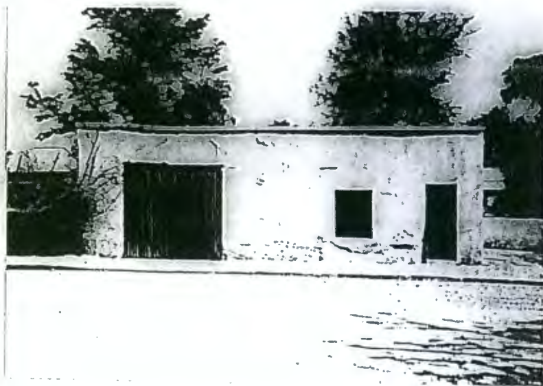
265. Erf ? (Old No. 0 1/2): Outbuilding, Bell Street.
