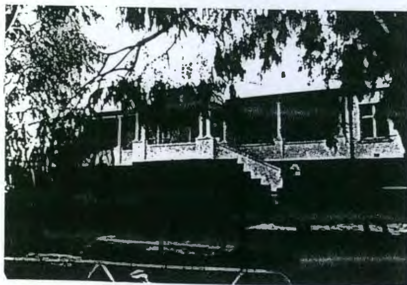
308. Erven 106 & 105: 10 West Church Street (facade faces Hofmeyer Street).
