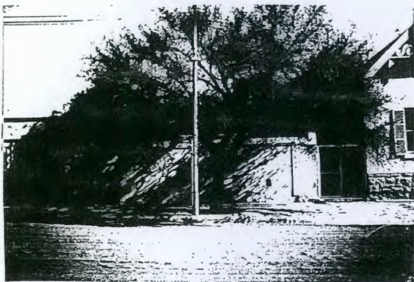
55/56. Erven 768/449: Wall between 3 & 5 d'Urban Row.
