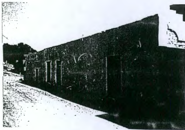
198. Erven 195, 196 & 197: Side facade of 27 Murray Street.
