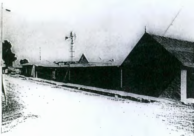
148. Erf 506: Back wall of 64 Church Street.
