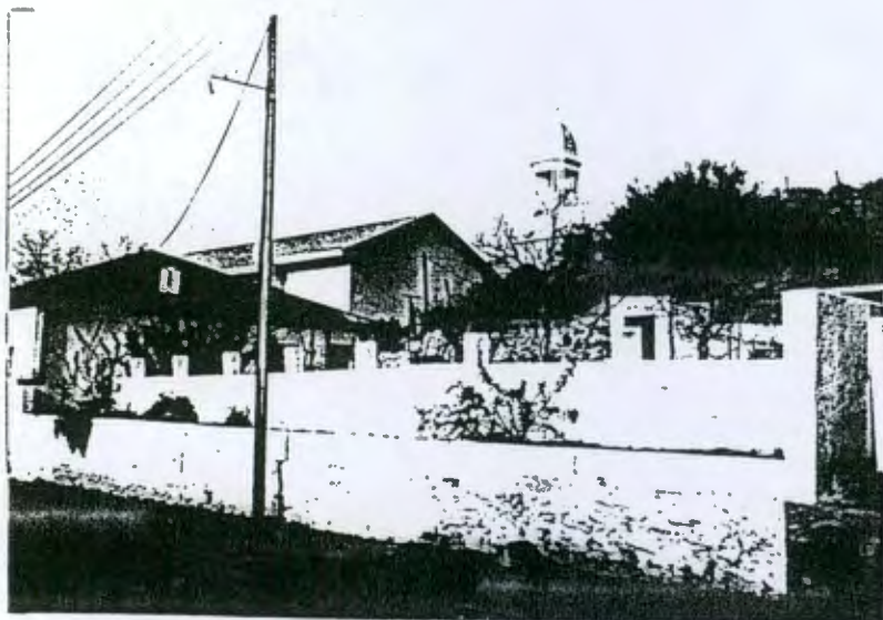
298. Erven 294 & 293: Wall of vacant lot, ? Bell Street.
