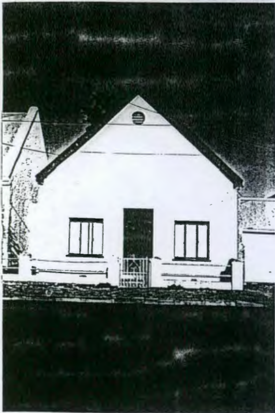
53. Erf 397: Methodist Church Hall.
