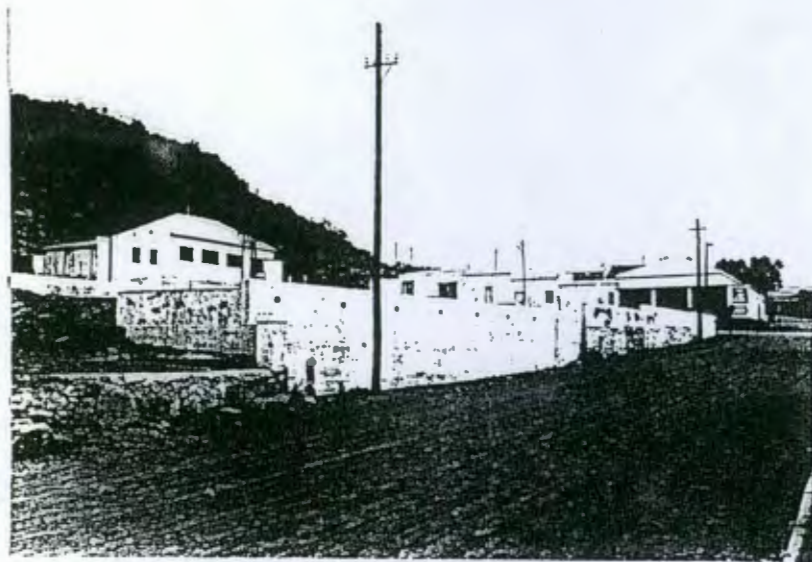
161. Erven 547, 548 & 549: Old wall, Campbell Street.
