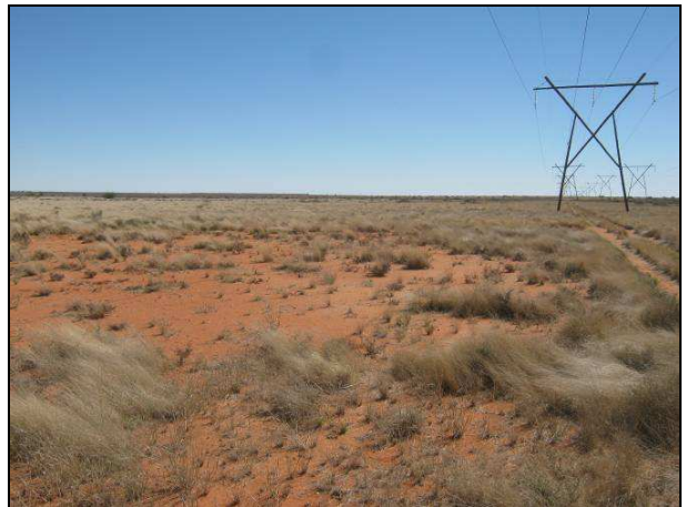
Figure 6: Sandy area and existing power lines along the southern edge of the site.
