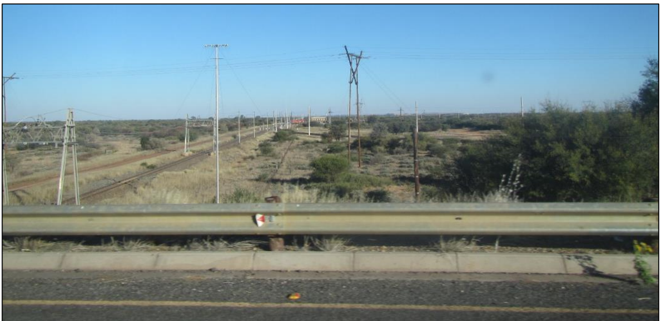
Figure 3: View towards the south from the road bridge over the railway showing infrastructure already present in the area.
