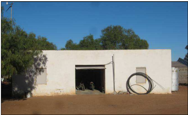
Figure 71: The outbuilding at SMS2012/001 (point 026).
