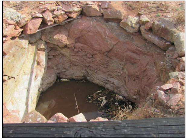
Figure 65: The 'putse' at KOE2012/003 (L086) located in Springbokvlei. Note the rock through which the well has been excavated.
