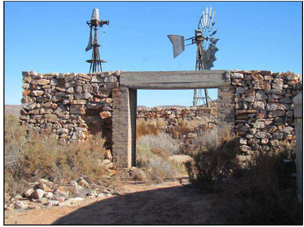
Figure 74: Ruined outbuilding at ARB2012/018 (point L054).
