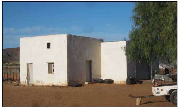
Figure 72: Second outbuilding at SMS2012/001 (point 026).
