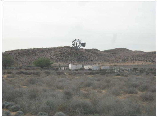
Figure 85: Water infrastructure at the Kangnas farm werf at KNG2012/001 (point 153).
