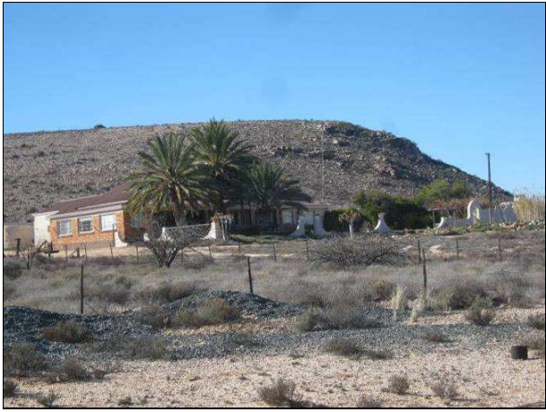
Figure 73: The main house at Areb (ARB2012/004; point 102).
