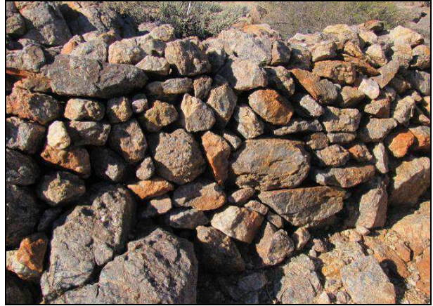
Figure 42: Close-up of the packed stone wall at SMS2012/002 (point 027).
