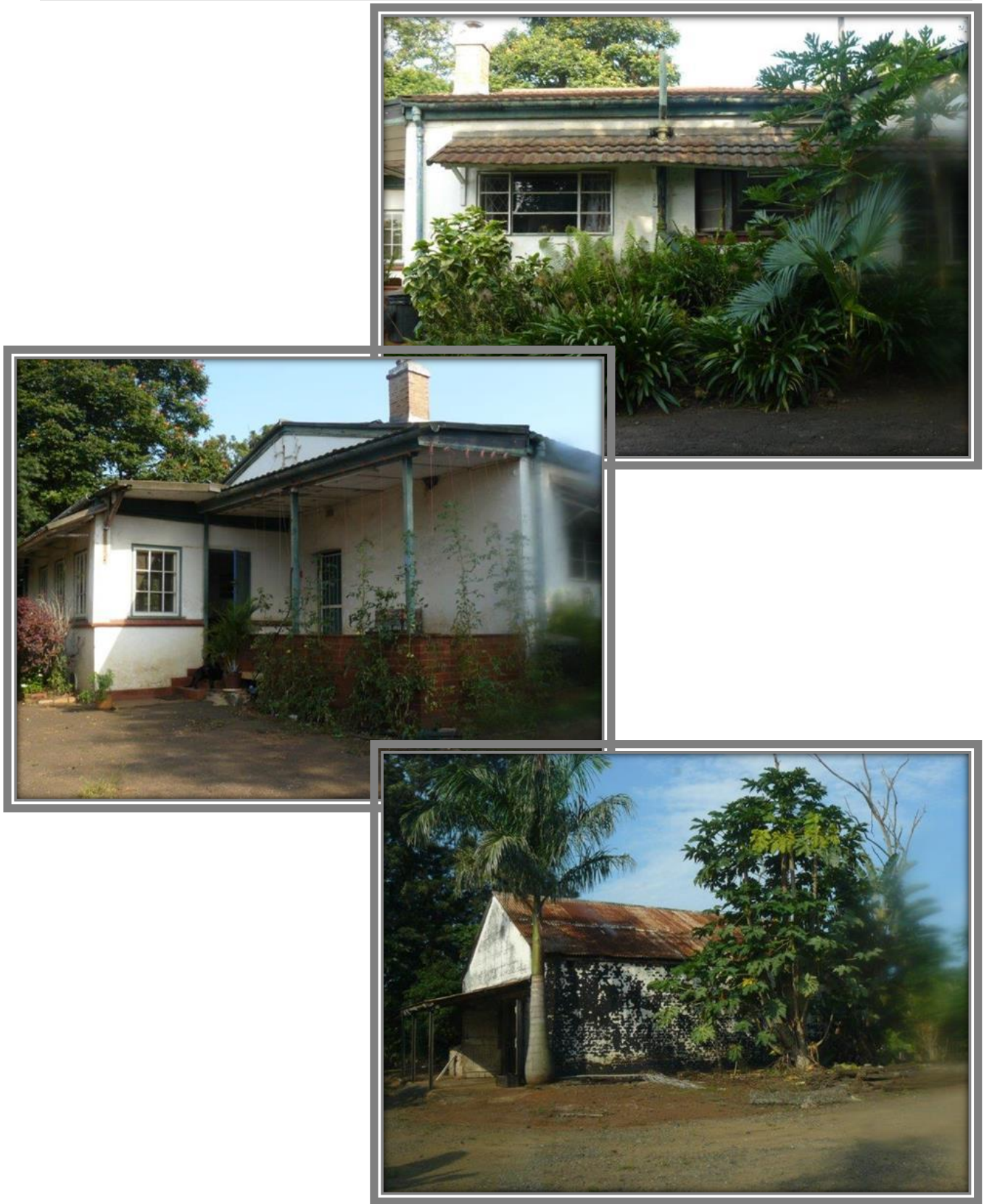
FIGURES 8-16 VARIOUS VIEWS OF THE FARMHOUSE WITHIN THE PROPOSED DEVELOPMENT SITE.
