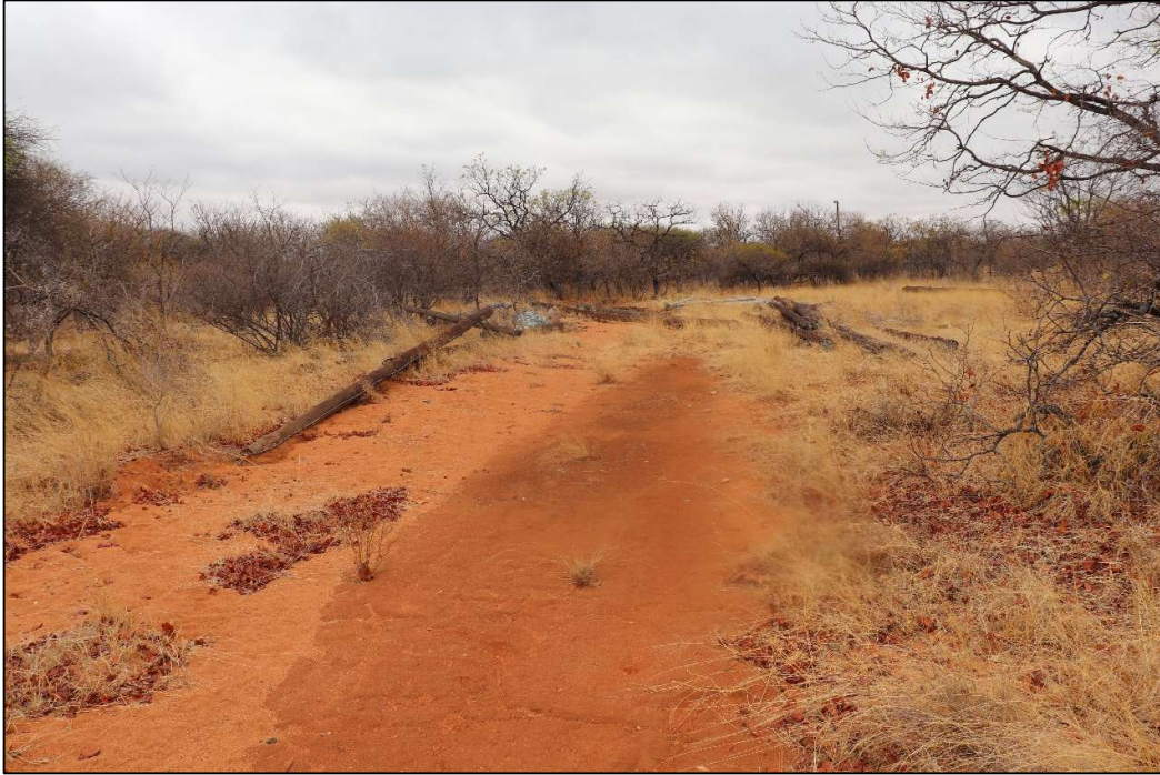
Figure 19: Abandoned gravel road leading to the earth dam, currently used to pile electrical poles
