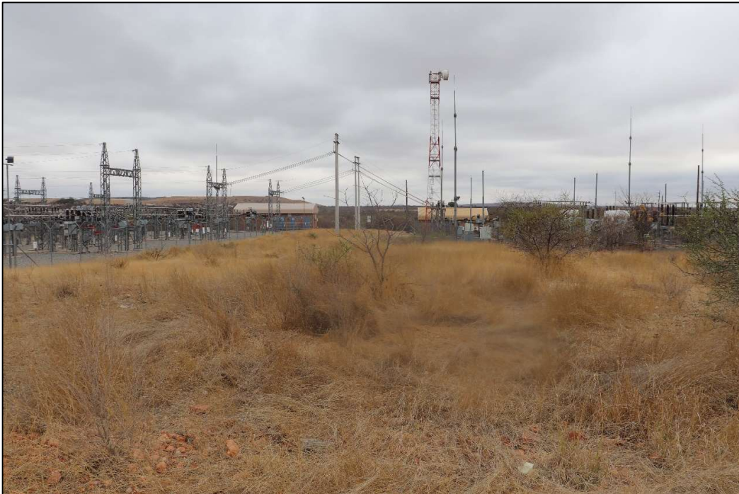
Figure 17: View of the substation
