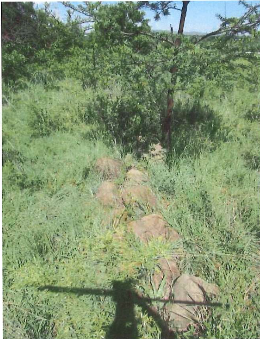
Figure 10: Section of the stone wall boundary at the grave site.
