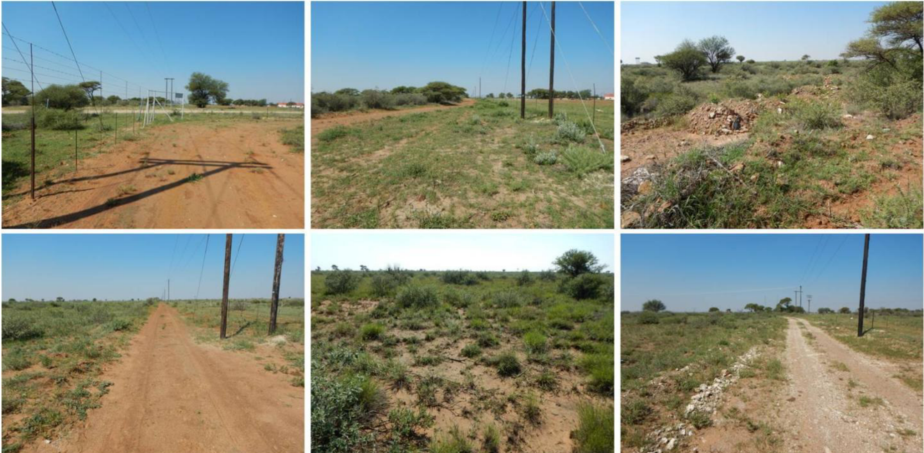
Plate 5. Examples of the affected environment along the overhead power line grid connection route showing flat terrain, mainly low and open vegetation with occasional trees, exposed ground surfaces and gravels, recent earthmoving activities (top right), single vehicle gravel tracks, overhead power lines and fencing.
