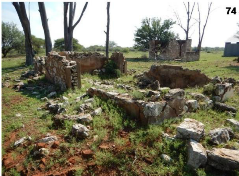
Plate 14. Structures at waypoint 74 include a small old cooler room (“fridge”) and calcrete structures in various stages of ruin. Note modern cement plaster in places while the mortar is clearly old and consists of local sediments.
