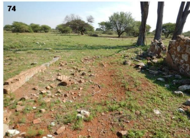
Plate 14. Structures at waypoint 74 include a small old cooler room (“fridge”) and calcrete structures in various stages of ruin. Note modern cement plaster in places while the mortar is clearly old and consists of local sediments.
