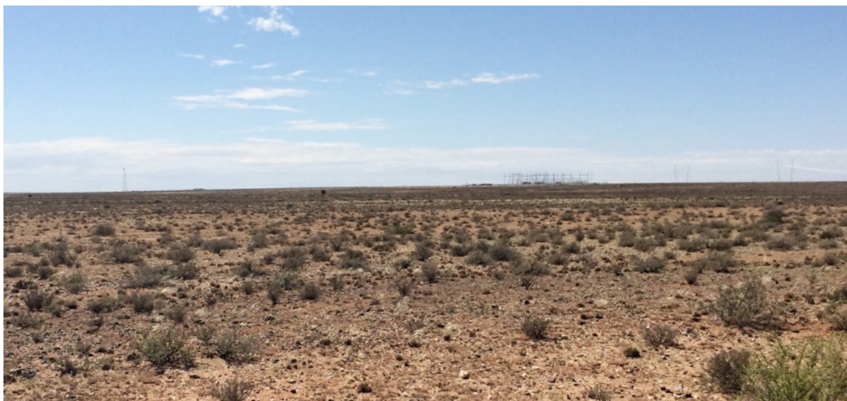
Figure 2120: Photograph 3 taken in a south-easterly direction along the proposed power line routing towards the existing Eskom substation, power lines and the cell tower.
