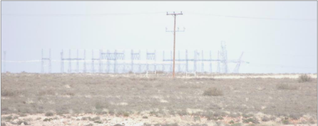
Figure 10: View of existing Cuprum substation
