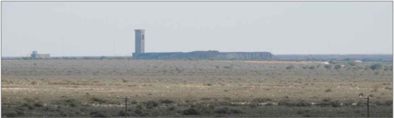
Figure 8: View of Copperton Mine headgear and Waste Rock Dumps as seen from the site
