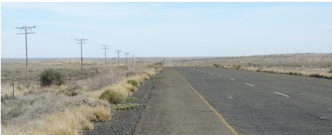
Figure 12: View east of the tarred section of the R357 road
