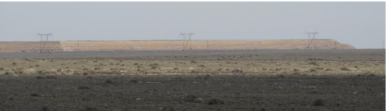
Figure 9: View of Copperton Mine Tailings Storage Facility as seen from the site
