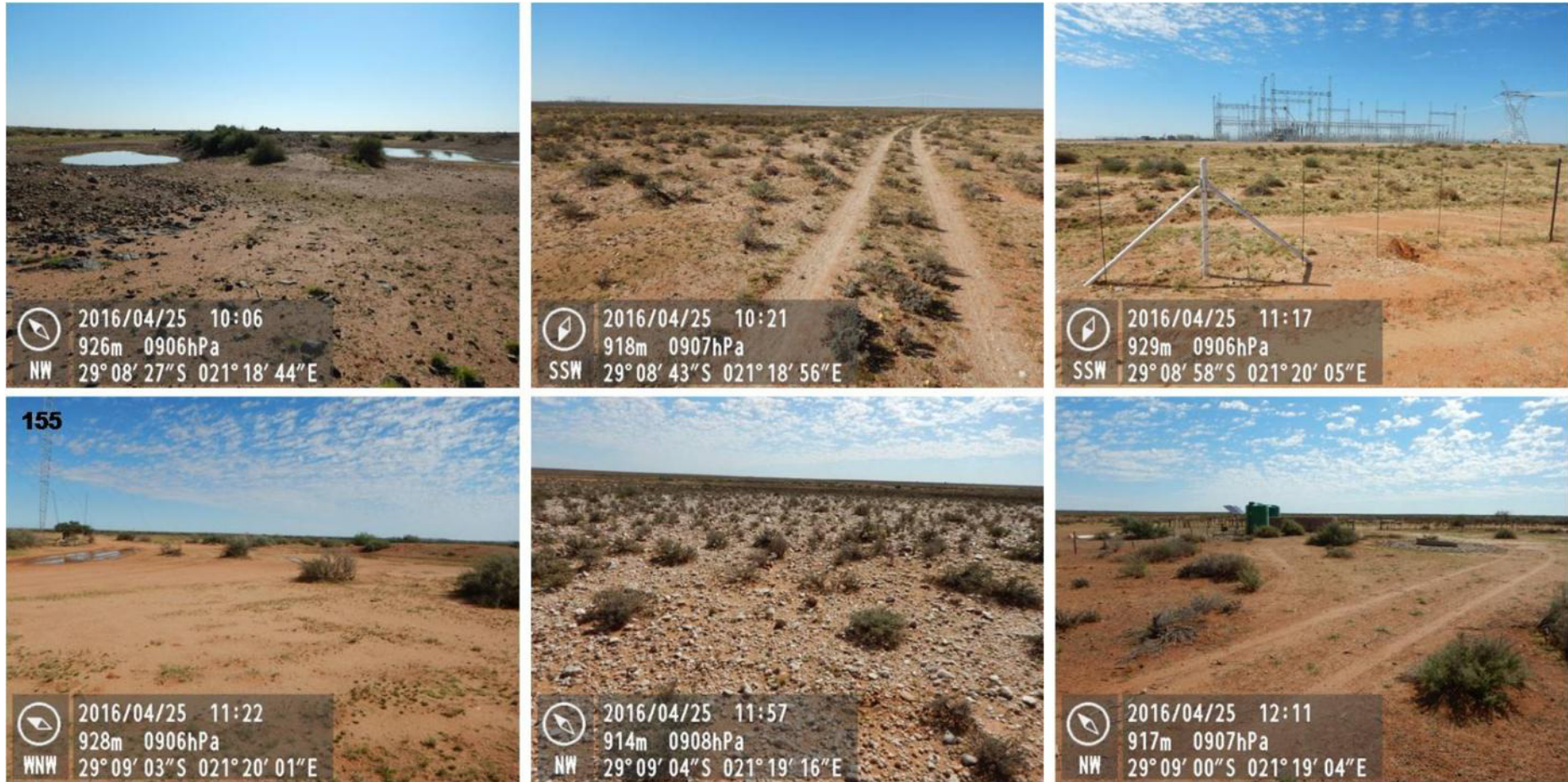
Plate 6. Examples of the affected environment along the overhead power line grid connection route showing recent earthmoving activities, vehicle track, the Nieuwehoop MTS sub-station, disturbed pan site at locality 155 (bottom left), exposed ground and quartz dominated gravels, flat terrain, low and open vegetation and recent developments including bore hole, free-standing cement dam, fencing, plastic water tanks, and watering and feeding troughs for domestic stock.
