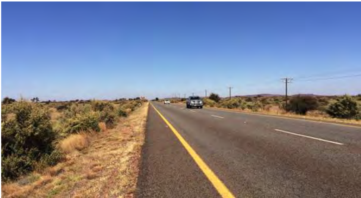
Figure 9: Photograph in a southerly direction of the N14 National Road
