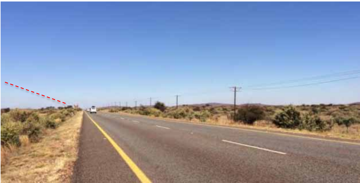
Figure 34: Photograph depicting the view south from the N14 road with the proposed alternative power line routed east of the road.
