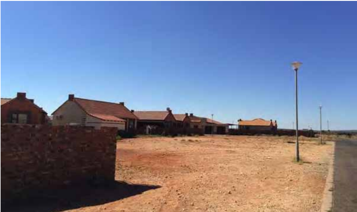
Figure 13: Photograph of the existing residential dwellings of the Bestwood estate.
