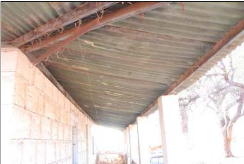
Figure 21: Corrugated iron roof sheets
