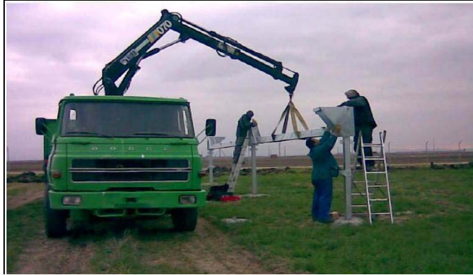
Figure 2.7 Mounting of the frame for the PV panels (Courtesy of Igeam, 2011)
