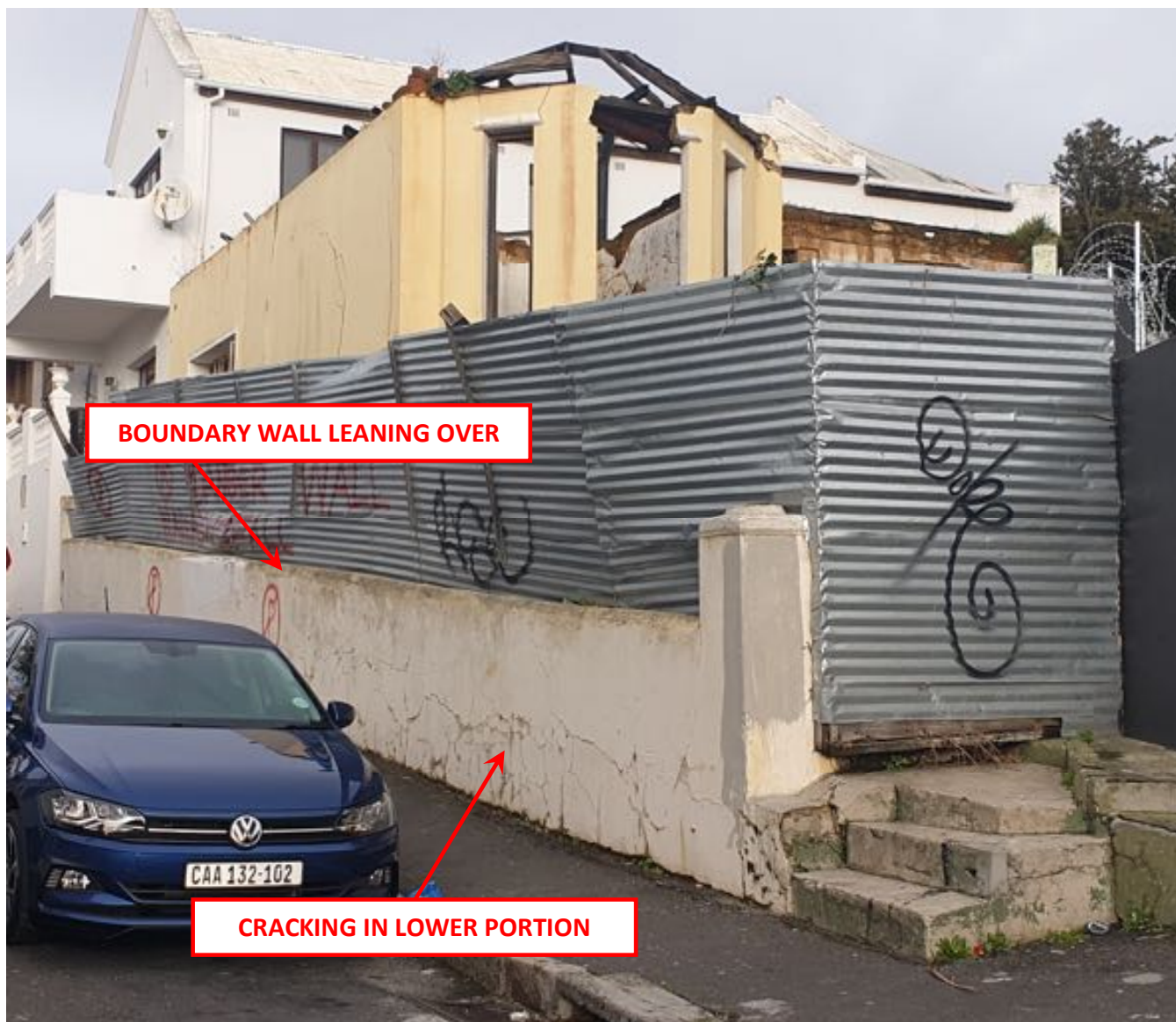
PHOTOGRAPH 7: STREET BOUNDARY WALL
