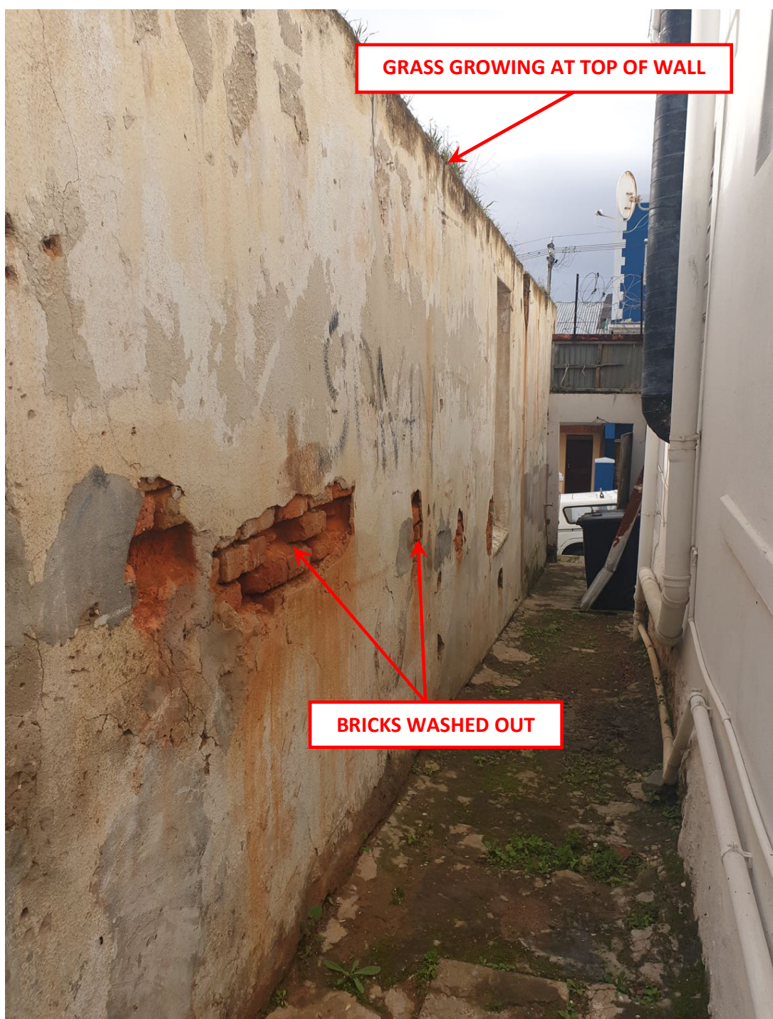
Photograph 2: EXTERNAL WALL ON BACK BOUNDARY
