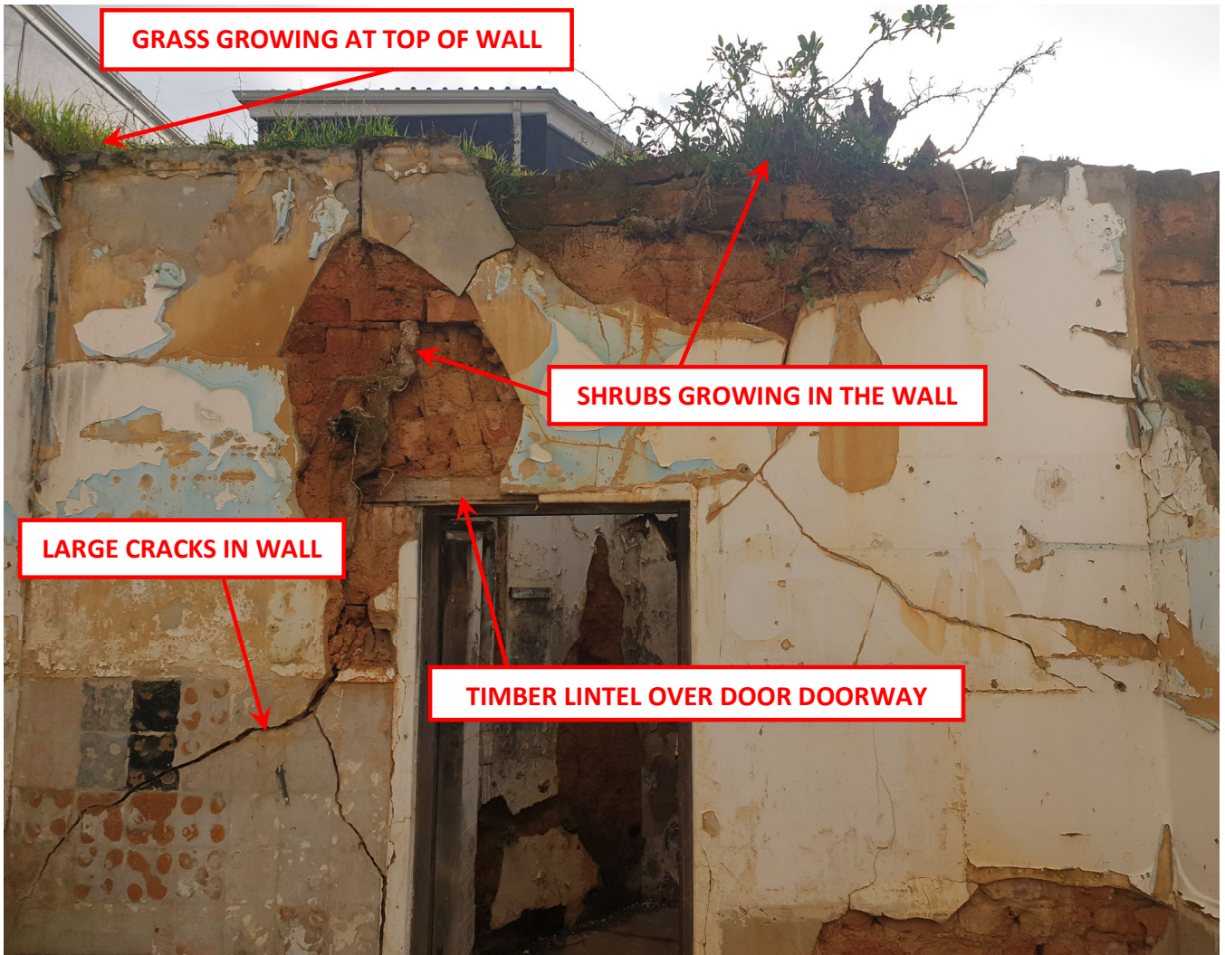
PHOTOGRAPH 3: WALL PANEL WITH DOOR OPENING
