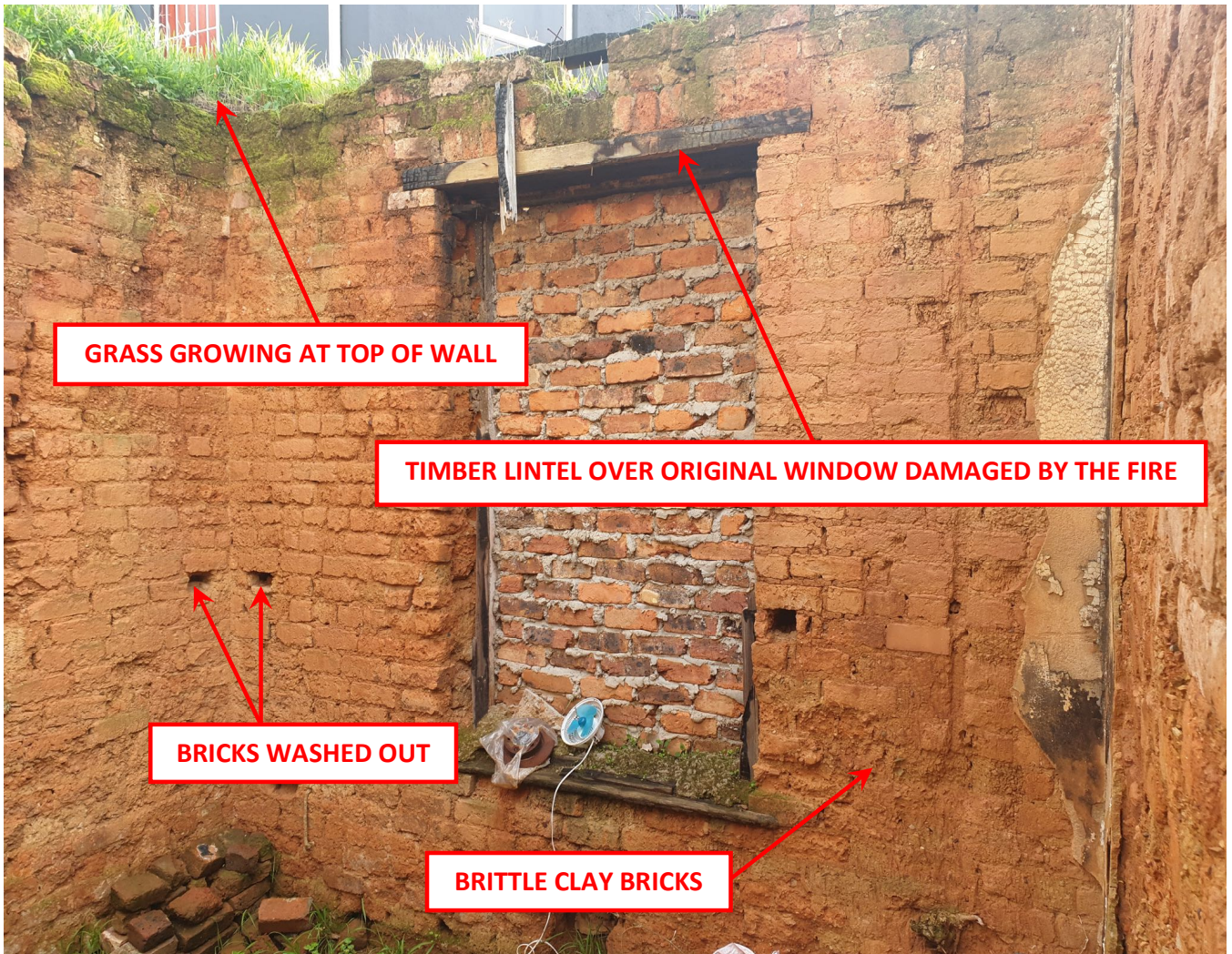
PHOTOGRAPH 4: ORIGINAL WINDOW CONSTRUCTION
