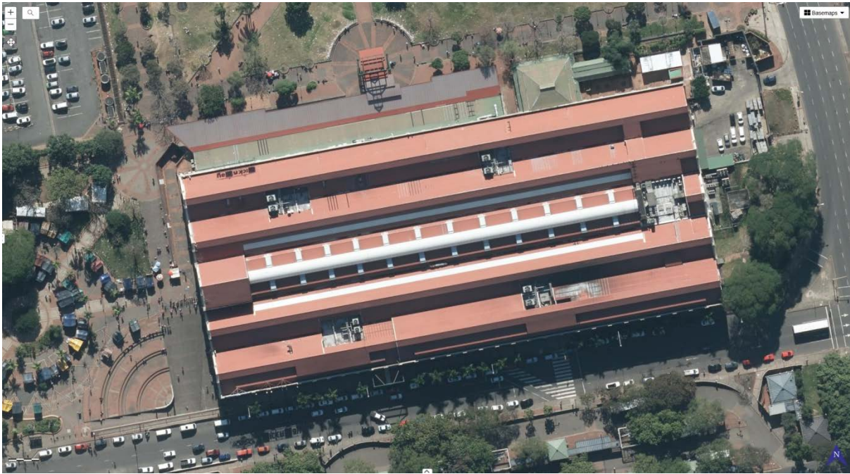
Existing Roof structure showing Polycarb sheeting
