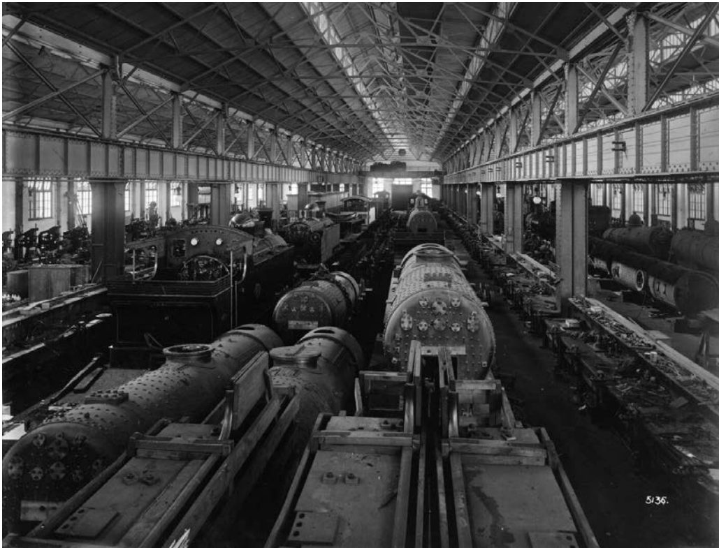
https://atom.drisa.co.za/ P1289-01.jpg – Internal Locomotive Shed
