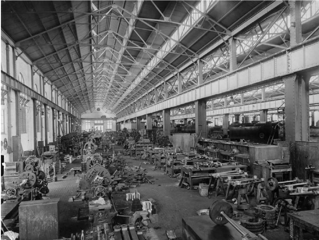
https://atom.drisa.co.za/ P1288.jpg – Internal Locomotive Shed
