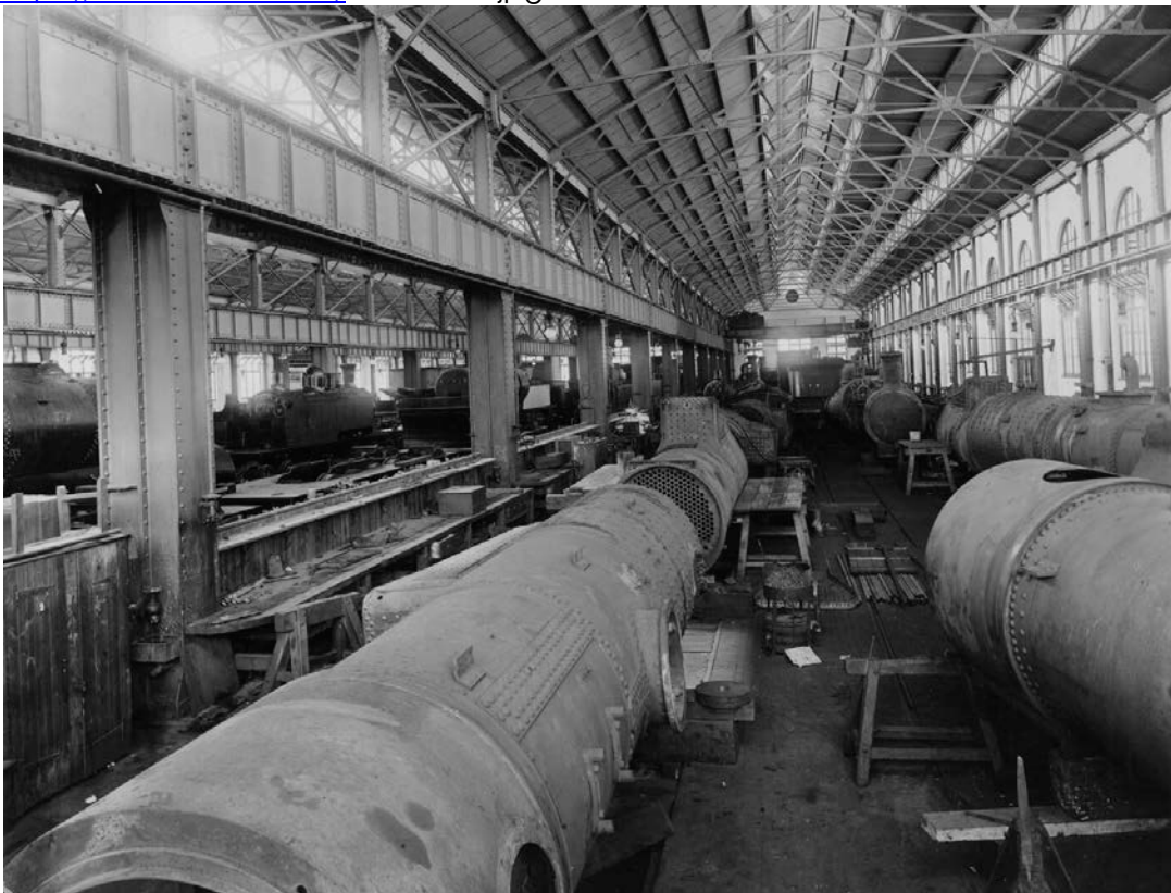
https://atom.drisa.co.za/ P1288-01.jpg – Internal Locomotive Shed
