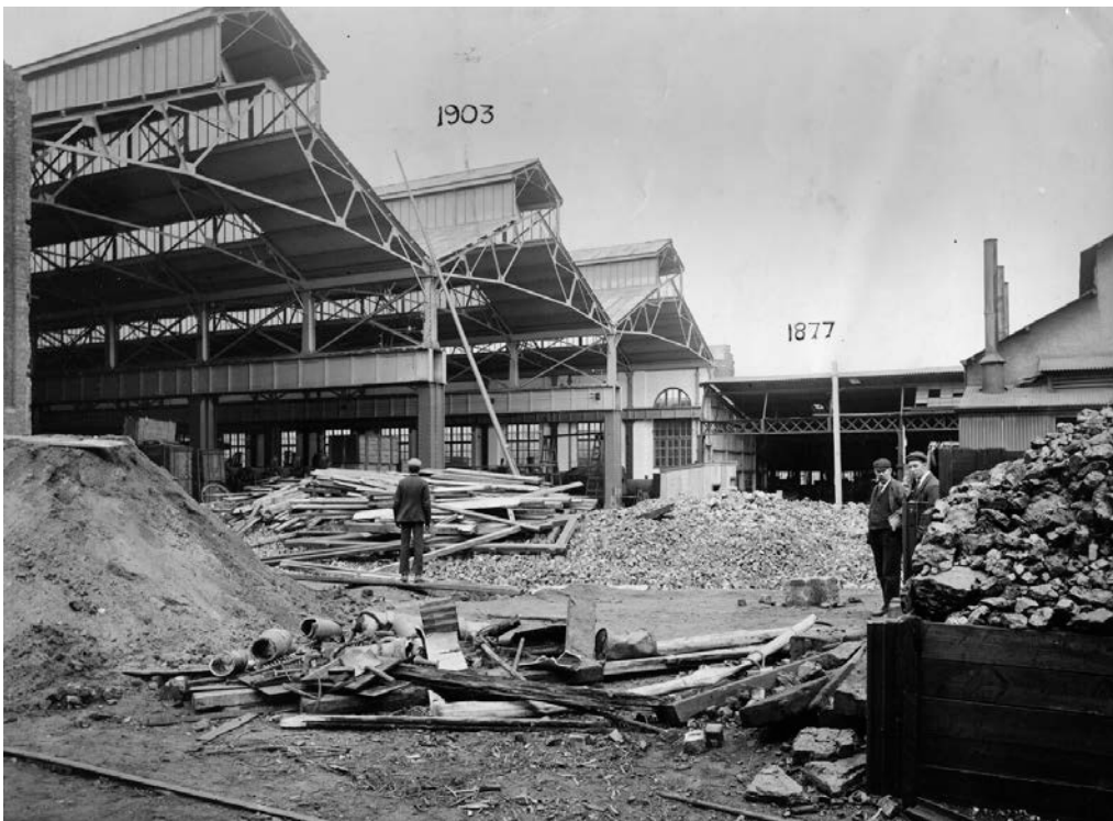
Relevant in showing steel structure, clerestory lighting and roof sheeting as well as columns and support beams
