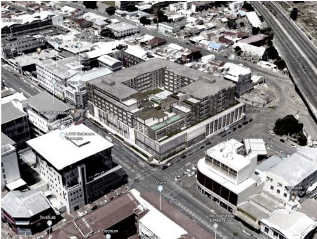
Figure 2.8: Aerial view of development from north-westerly direction
