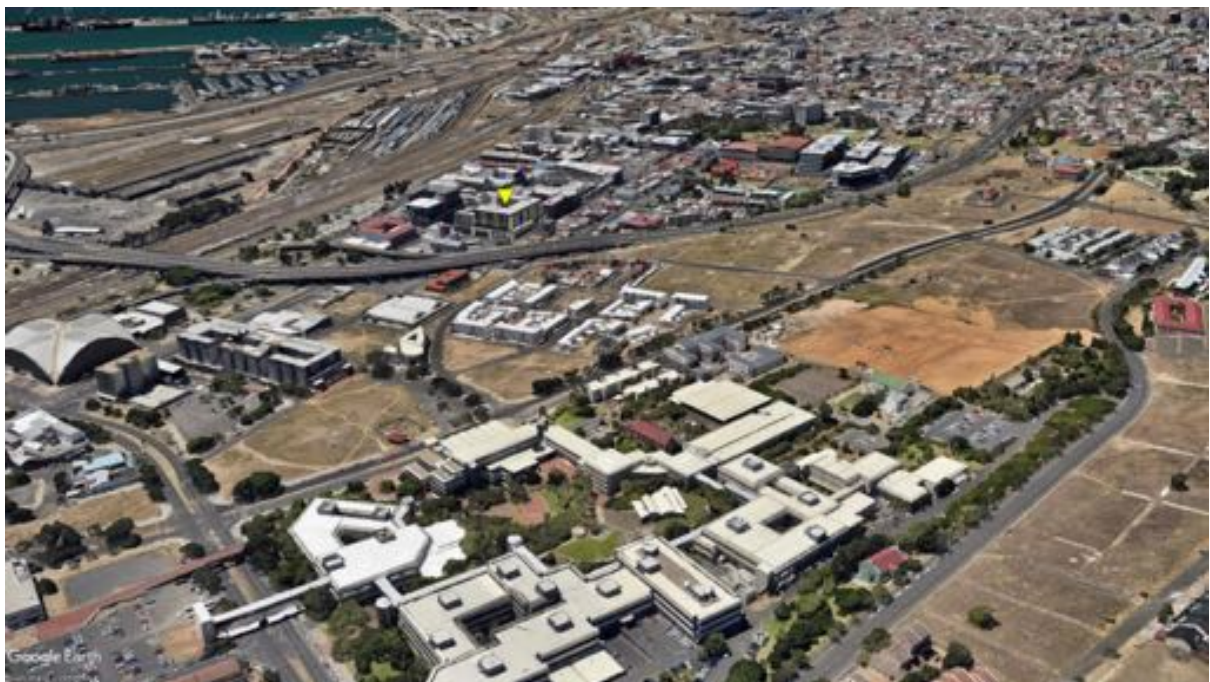
Figure 4.4: Birds-eye view from District 6 looking towards Woodstock, railways and harbour beyond Source: Adapted from Google Earth, 2020
