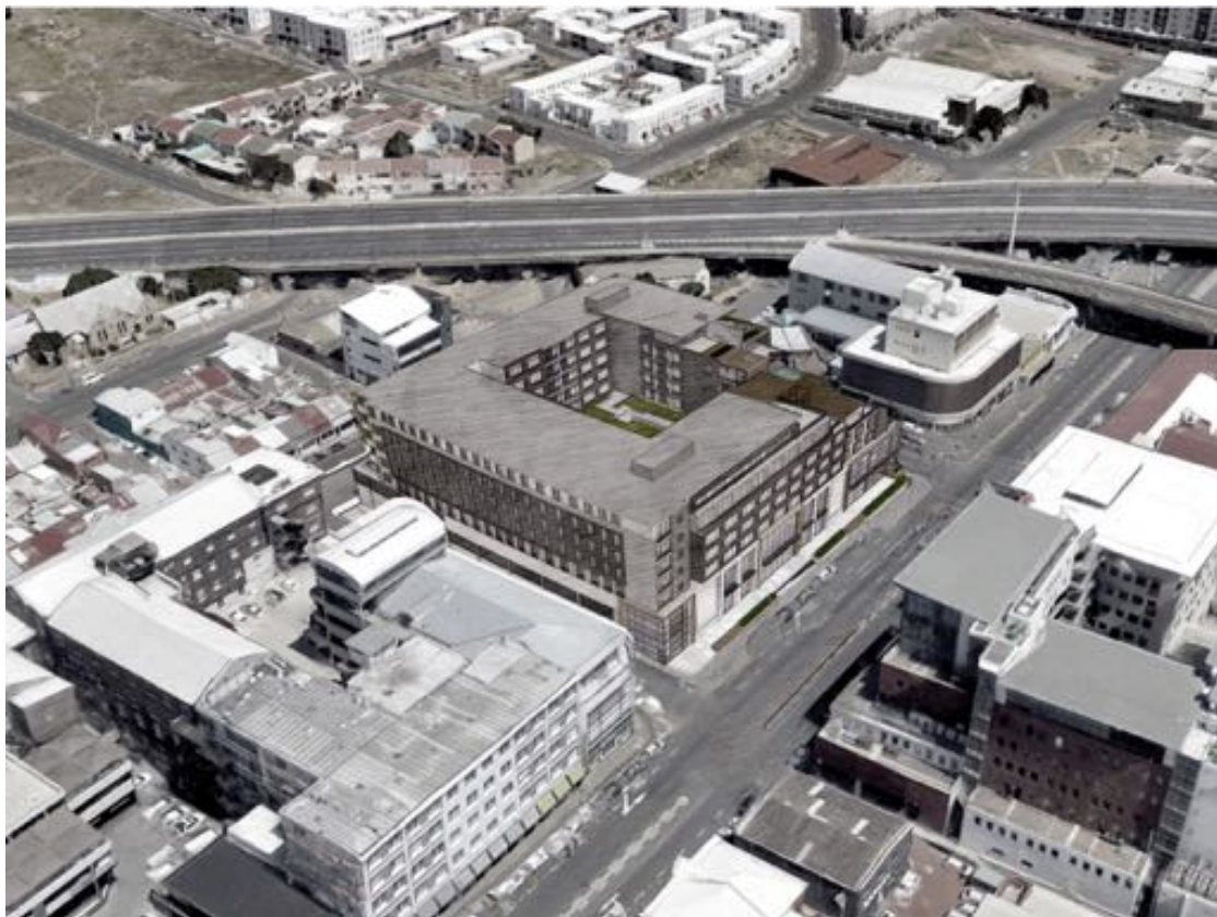
Figure 2.9: Aerial view of development from north-easterly direction
