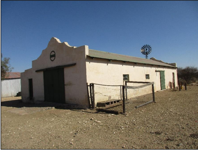
Fig 10. A shed at the farmstead.
