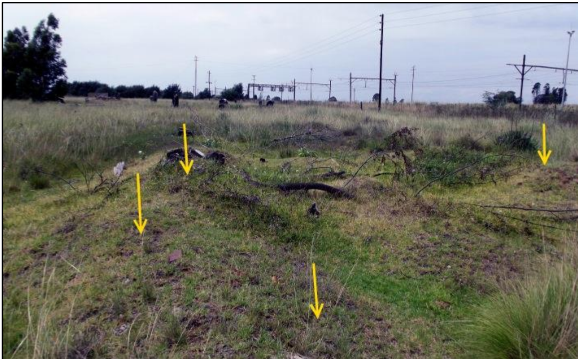
Fig. 8. Site PZ 6. The arrows show the demolished remains of a building or possibly a dwelling. Photos were taken in an eastern direction.
