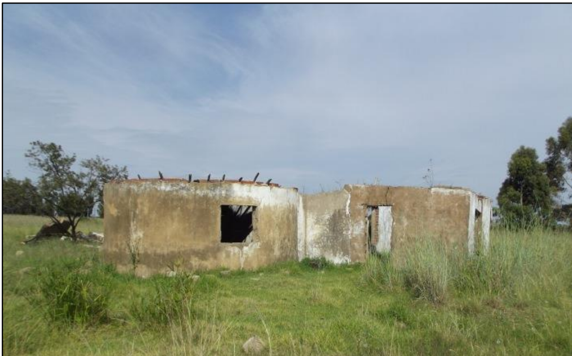
Fig. 2. Site PZ 1. Photo taken in western direction.
