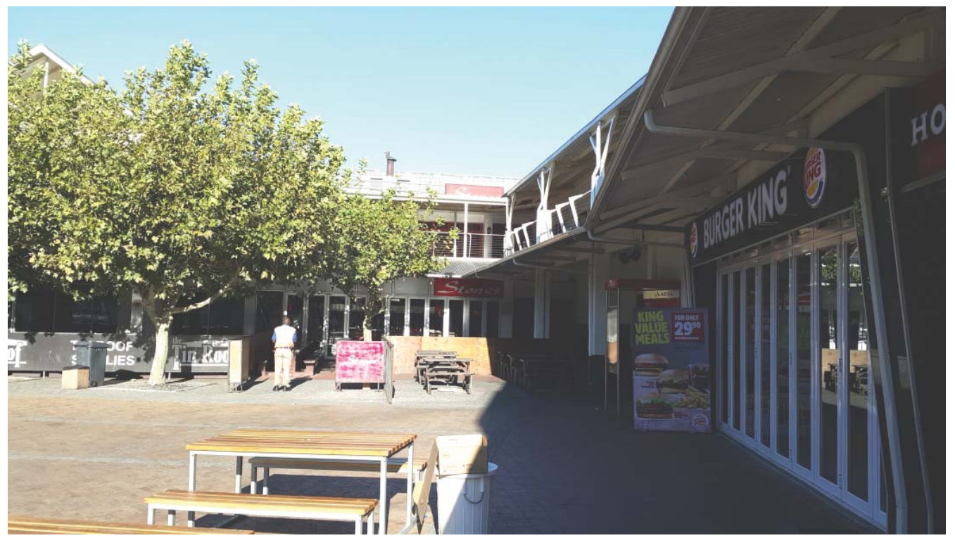
EXISTING BUILDINGS TO BE DEMOLISHED
