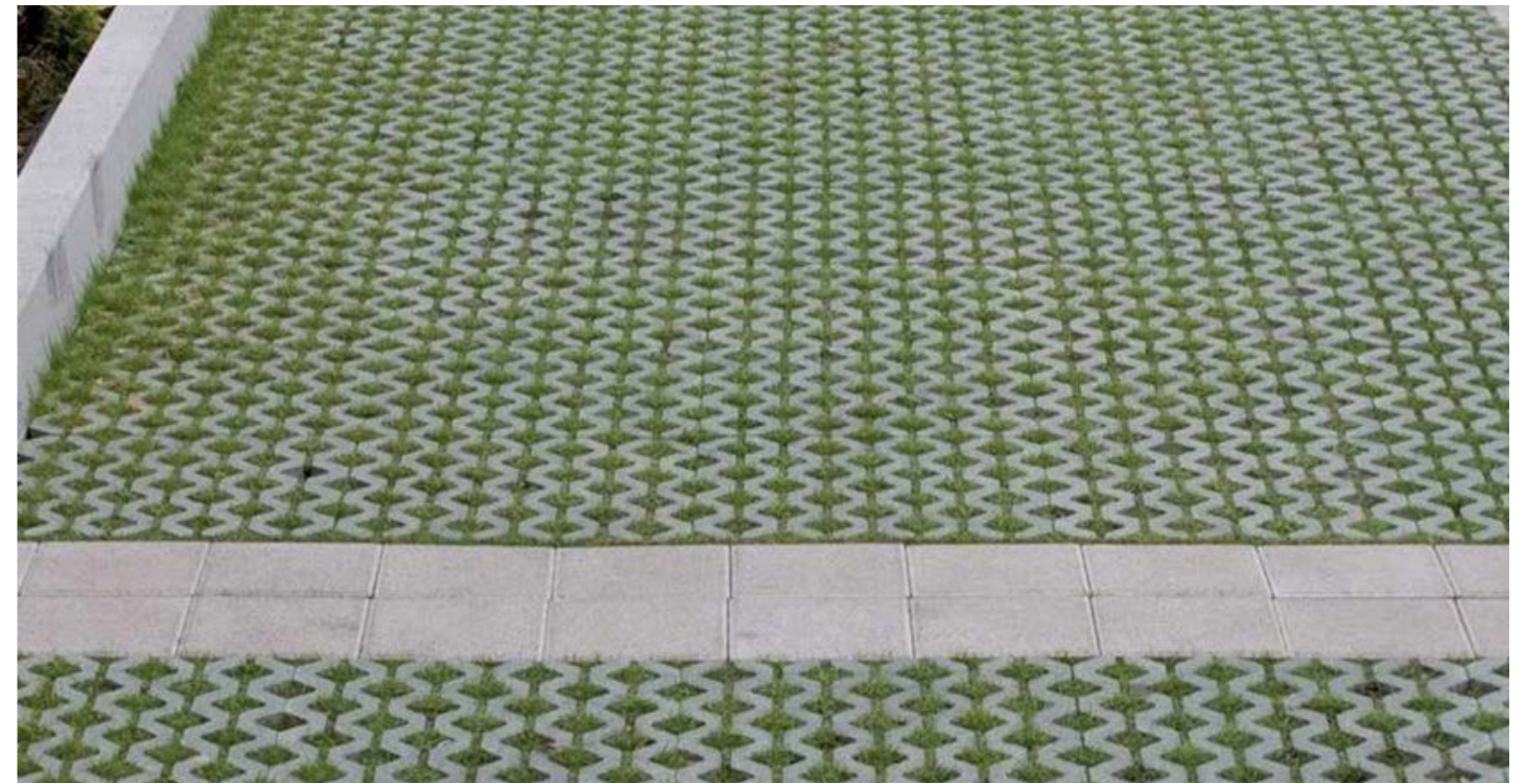
Permeable paving with grassblocks with paving accents
