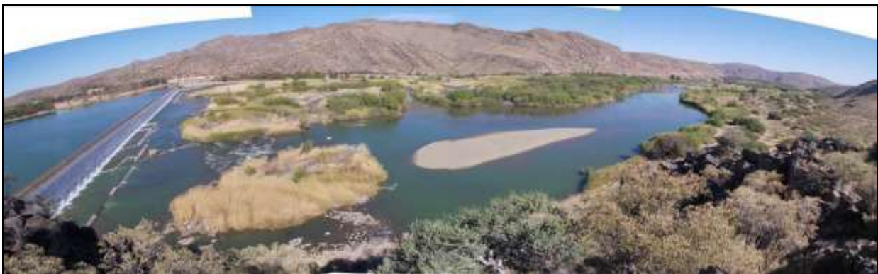
Figure 2: View from above the Boegoeberg weir showing the character of the river valley at this point. The photograph is taken from the top of the small cliff below which the power station would be built.
