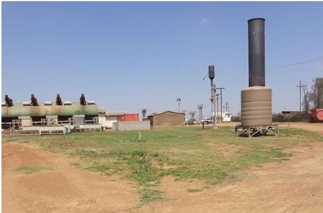
Fig. 22. Photo taken from position 14 in fig 11 covering proposed Desulphurisation CHP 1 & 2 and Gas cooling in fig. 10. (S.M.Miller September 2020.)
