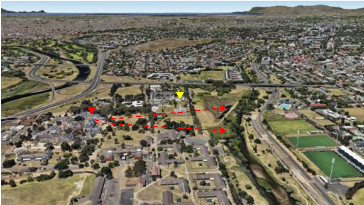
Figure 4.1.4: Bird’s-eye view of the proposed development in a southerly direction looking towards Rondebosch Common and the southern suburbs. (Google, 2022)
