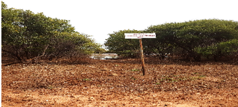
Fig. 14. The western side of OMWSD 4 is already naturally damming rainwater against the eastern wall of sludge dam OMWSD N&R. (Photo S.M. Miller 2021.)
