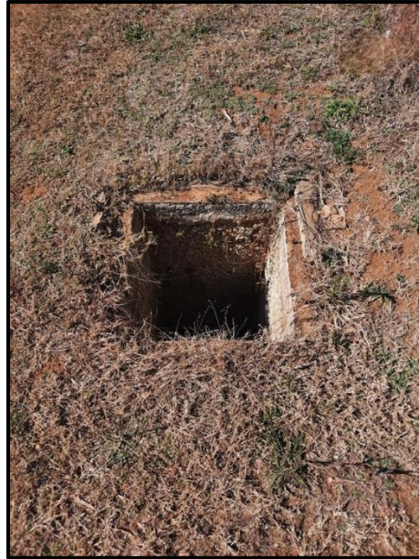
Figure 7.6. Manholes marking the existing sewage line.
