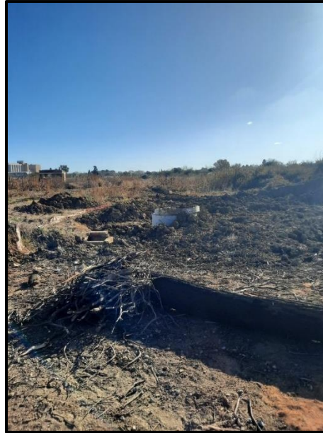
Figure 7.2. Portions of the Leeuwkuil project already under construction.
