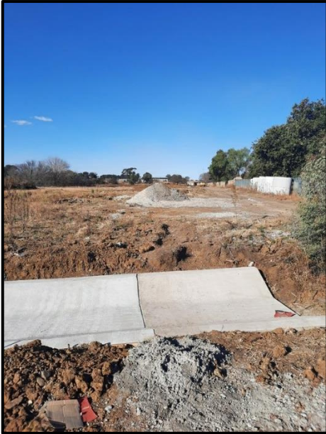
Figure 7.1. Portions of the Leeuwkuil project under construction.
