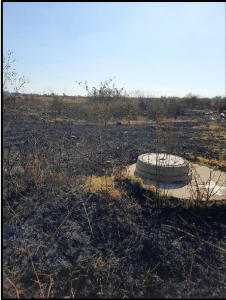
Figure 7.5. Existing sewage line marked by manholes.
