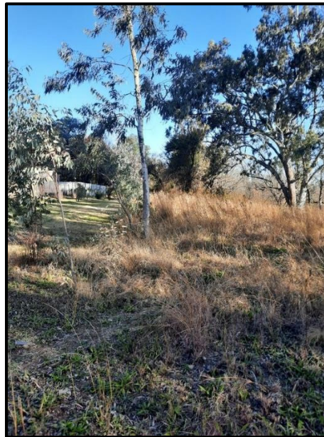
Figure 7.4. Pipeline alignment along the edge of a row of properties next to the Kliprivier.
