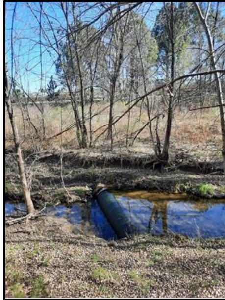
Figure 7.10. Existing sewage line within the Emerald Casino premises.
