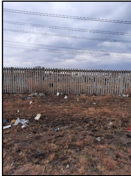
Figure 8.7. View of Vuka cemetery showing the existing fence.
