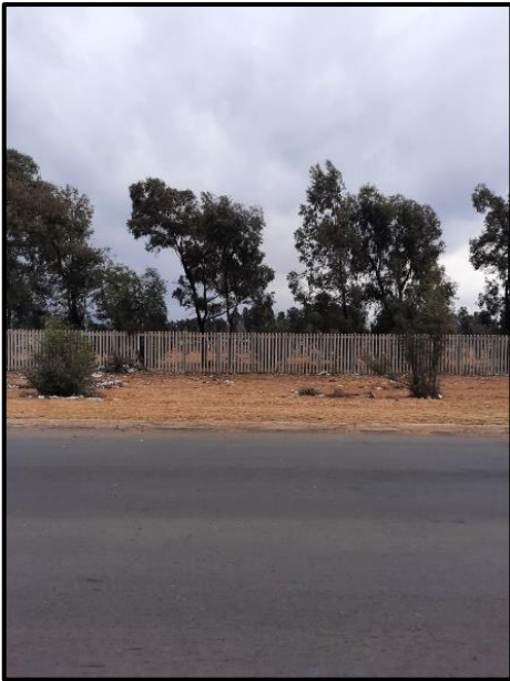
Figure 8.6. View of Vanderbijlpark cemetery from Andries Potgieter Blvd showing the existing fence.
