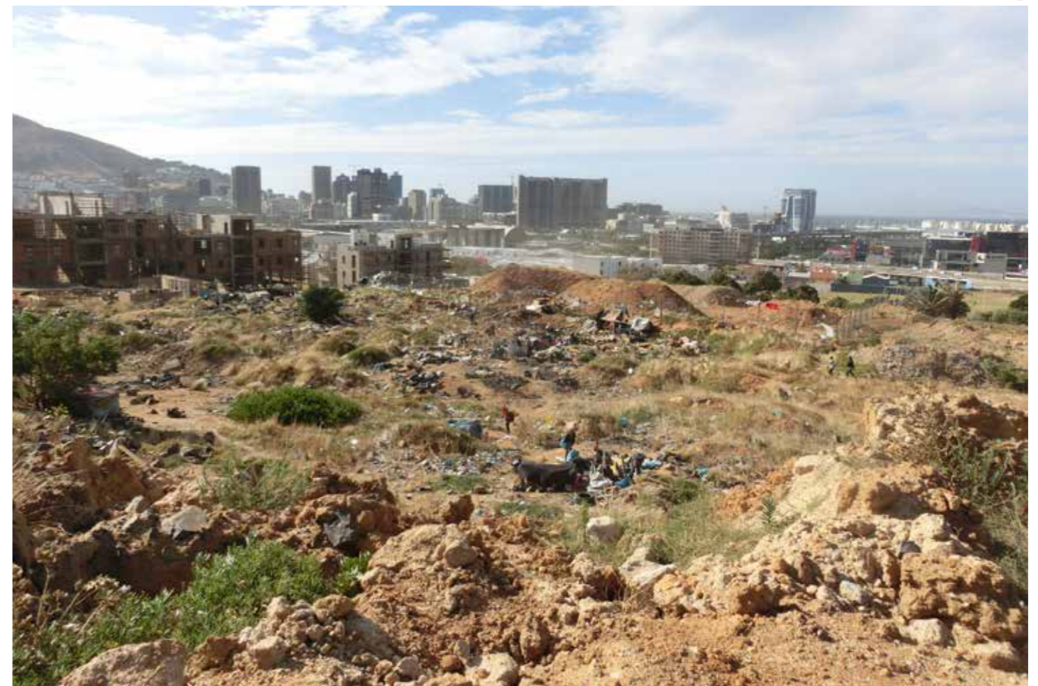
Figure 4. Phase 4 during site levelling, view to north (RSA, 2020)
