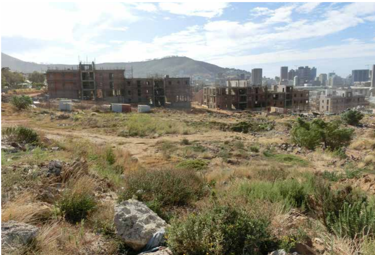
Figure 2. Phase 4 during site levelling, view to north west (RSA, 2020)
