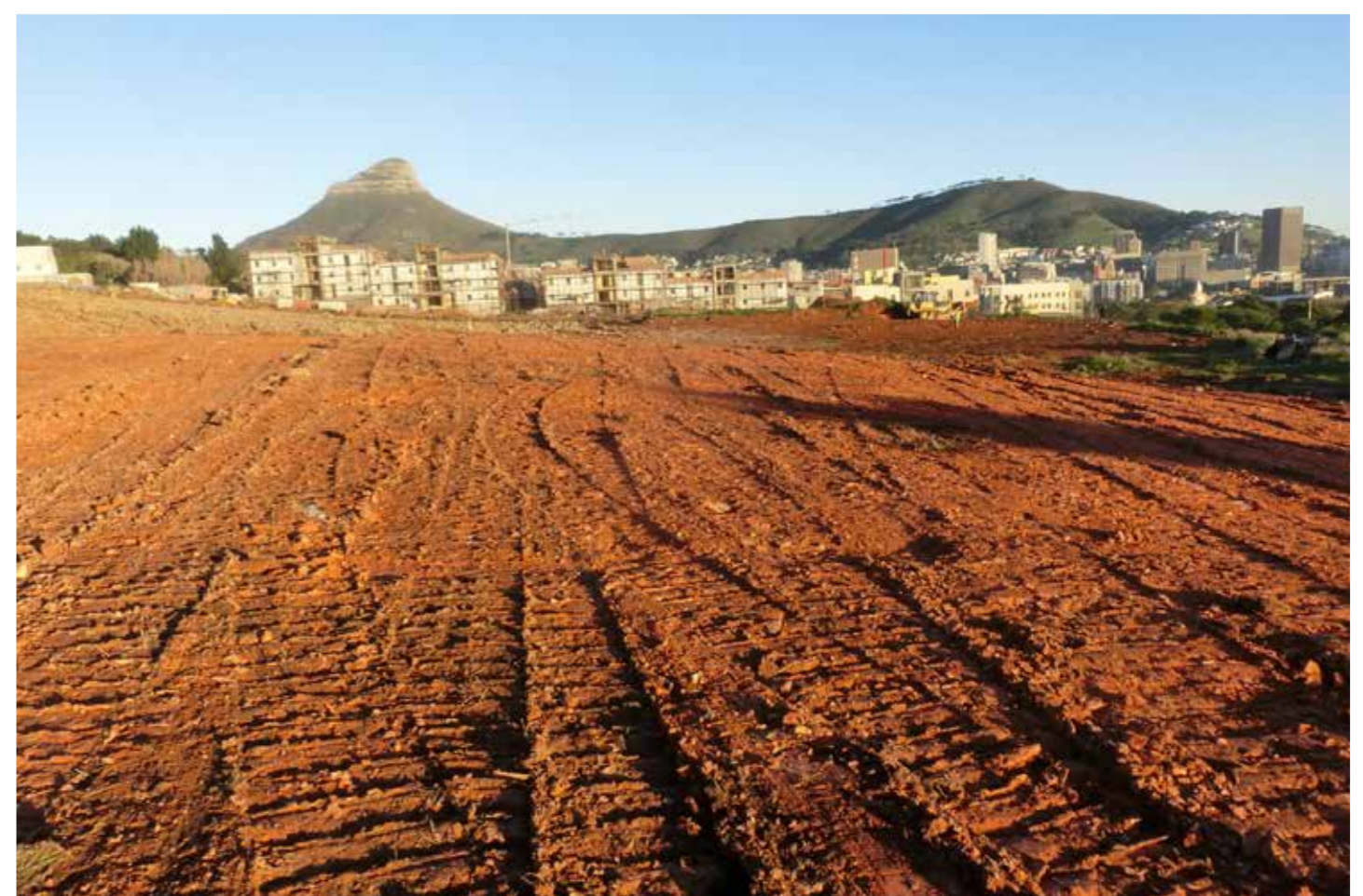
Figure 5. Phase 4 during site levelling, view to west (RSA, 2020)
