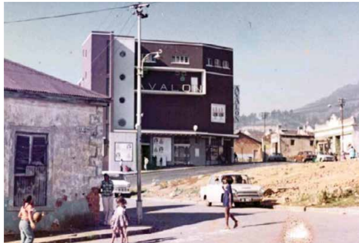
Figure 29. The Avalon Cinema exterior (top) and interior (below) (District Six Museum, 2022)
