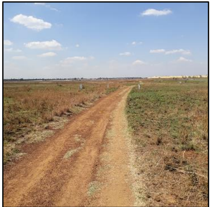
Figure 7. Road and pipelines
