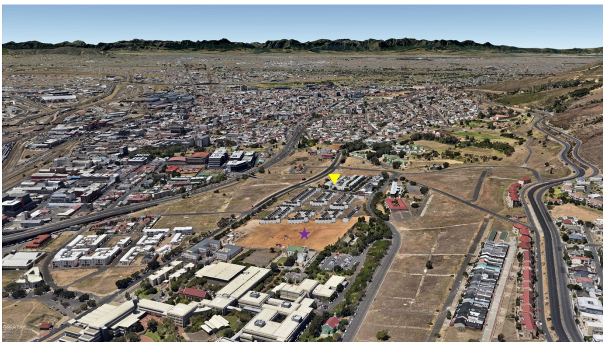
Figure 4.2.4: Birds-eye view of the proposed development from the CBD looking towards Woodstock and beyond. (Google; 2022)
