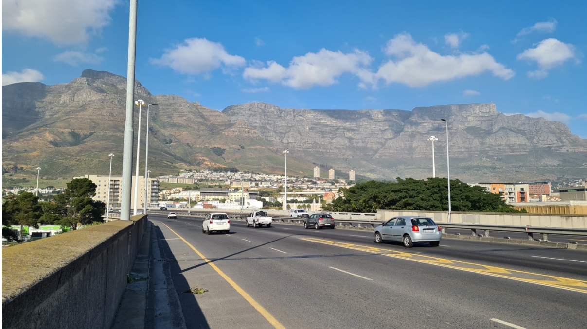
Figure 2.4.2: View along Nelson Mandela Boulevard. (SQ1, 2022)
