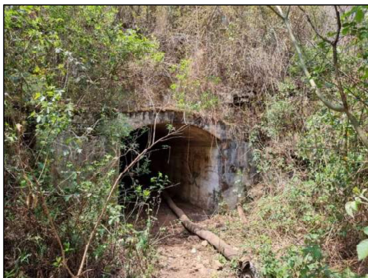
Figure 6-8: View of Historical / Extant Adit in the Beta North Mining Area.
