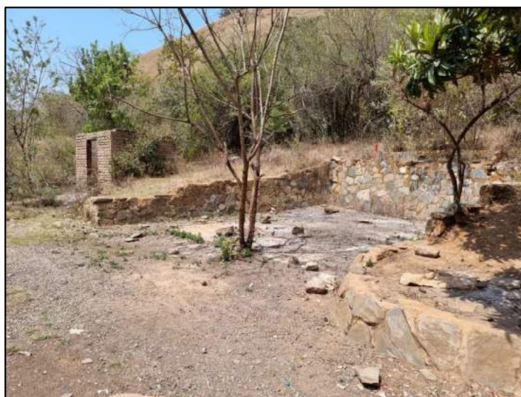
Figure 6-3: View of the dilapidated mining infrastructure in the Beta Mine area.
