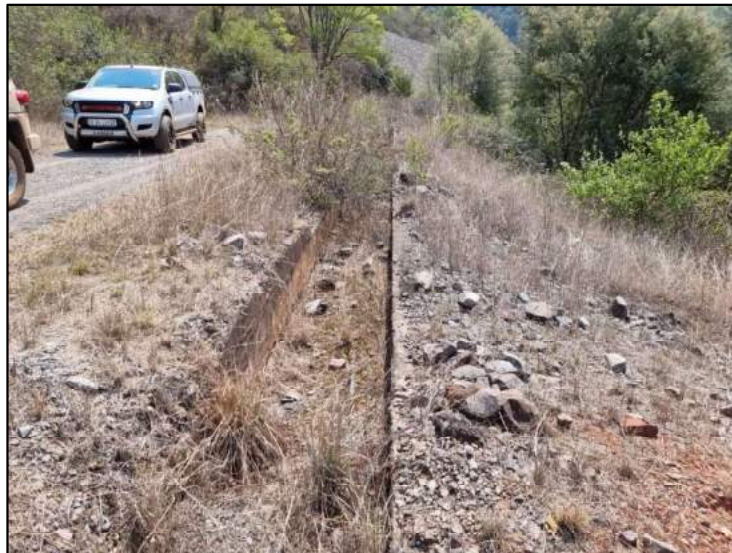
Figure 6-14: View of the partial remains of a Historical concrete water furrow in the Beta North Mining Area.
