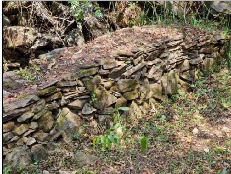
Figure 6-43: View of a stone wall feature at the extant Morgenzon/ Clewer adit.
