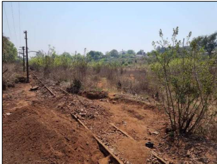
Figure 6-6: View of the dilapidated remains of the Historical tram line/cocopan line and power line posts in the Beta Mining area.
