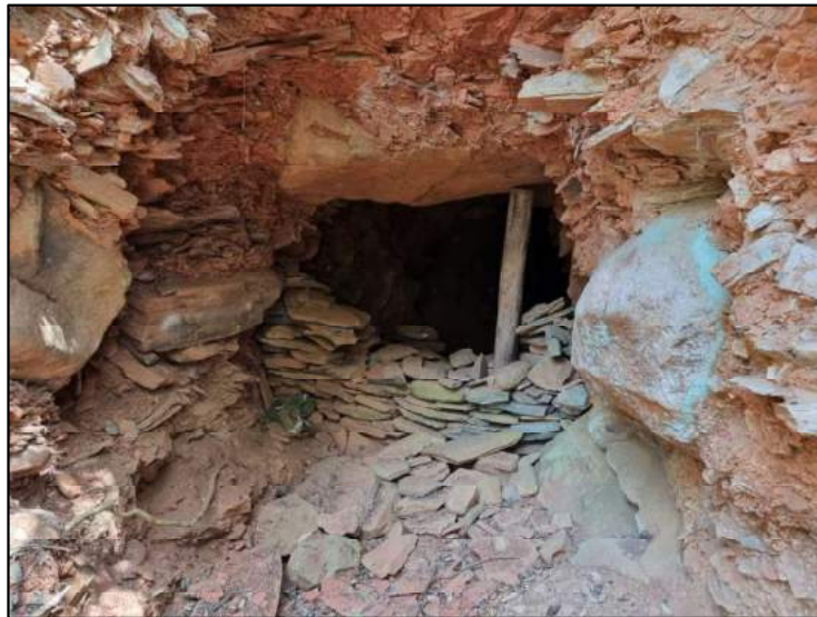
Figure 6-44: View of a ventilation shaft at the Morgenzon/ Clewer adit.
