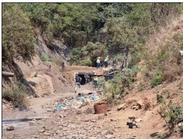
Figure 6-40: View of the extant Lower Dukes mine adit.
