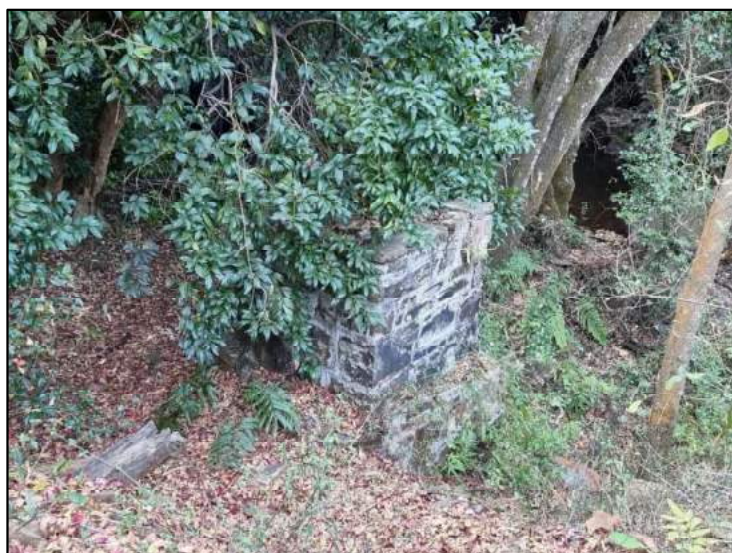
Figure 6-32: View of a stone support structure at NH-TGME-2430DC-11.
