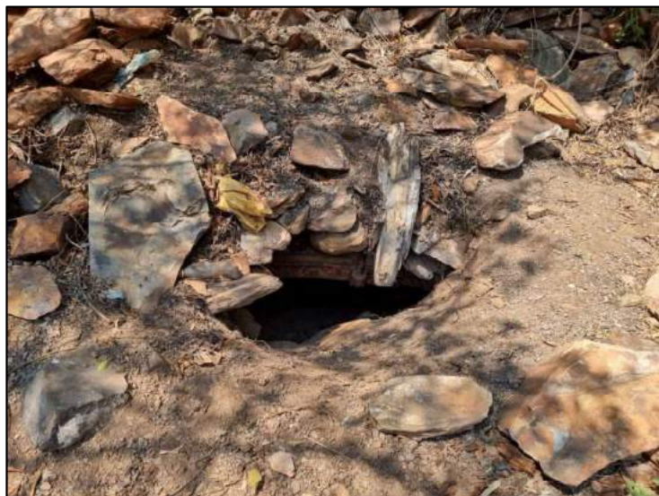
Figure 6-39: View of a collapsed Historical Adit in the CDM Mining Area at the Lower Dukes mine.
