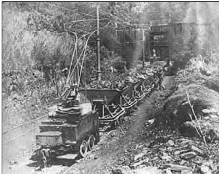
Figure 6-13: A historical image of the Historical tram line / cocopan line and power lines in the project landscape.
