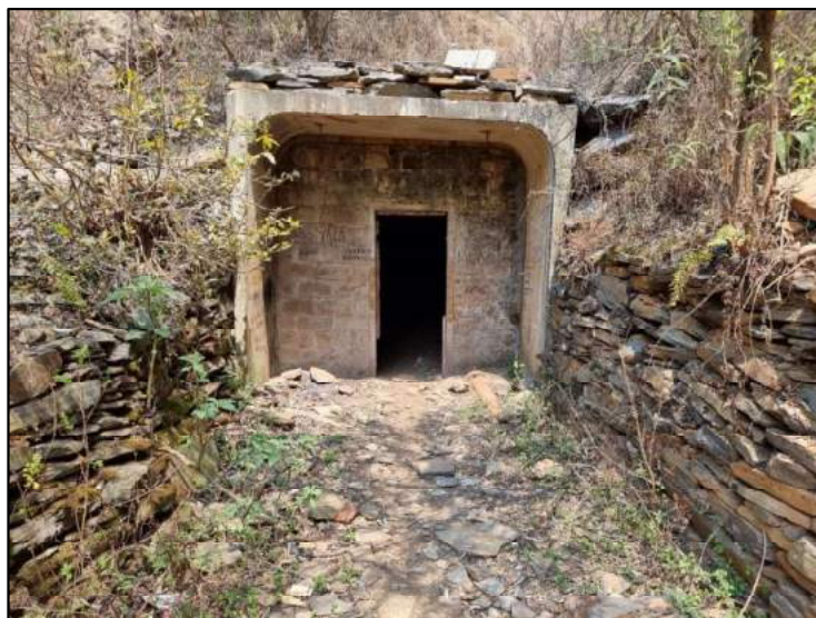
Figure 6-42: View of the extant Morgenzon/ Clewer adit. Note stone wall structures stabilizing the surrounding mountain slopes.
