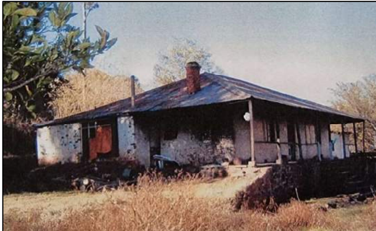
Figure 6-19: An archive photo of the mine manager's house dating to 2005 (Pistorius).
