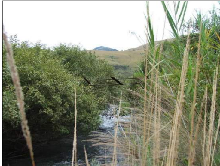
Figure 6-15: View of the remains of a Historical suspension bridge in the Beta North Mining Area (PGS 2008).
