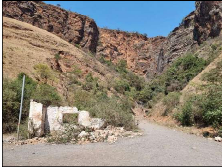
Figure 6-34: View of the dilapidated mining infrastructure in the CDM Mining Area at the Lower Dukes mine.
