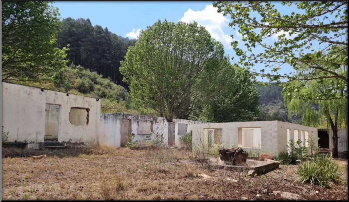
Figure 22: Neglected site of the Morgenson - mining Offices
