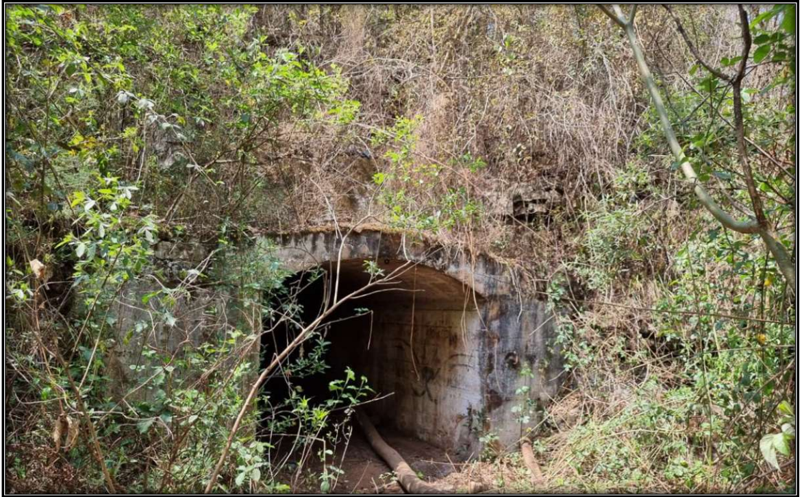
Figure 8: Adit at Beta North
