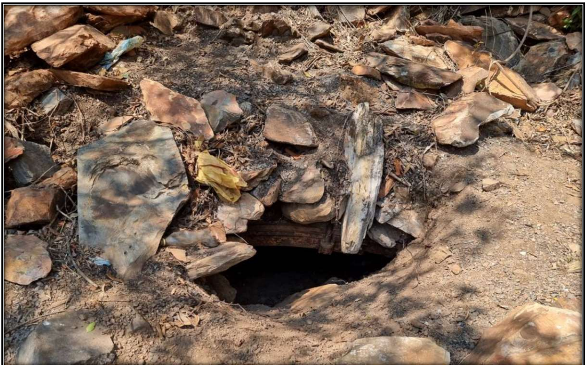
Figure 15: Vent shaft at Dukes mine.
