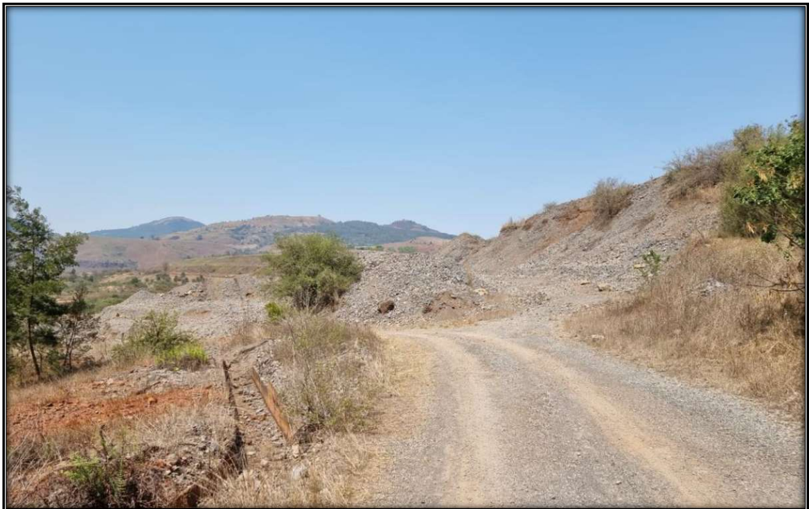
Figure 7: Access Road to Beta North
