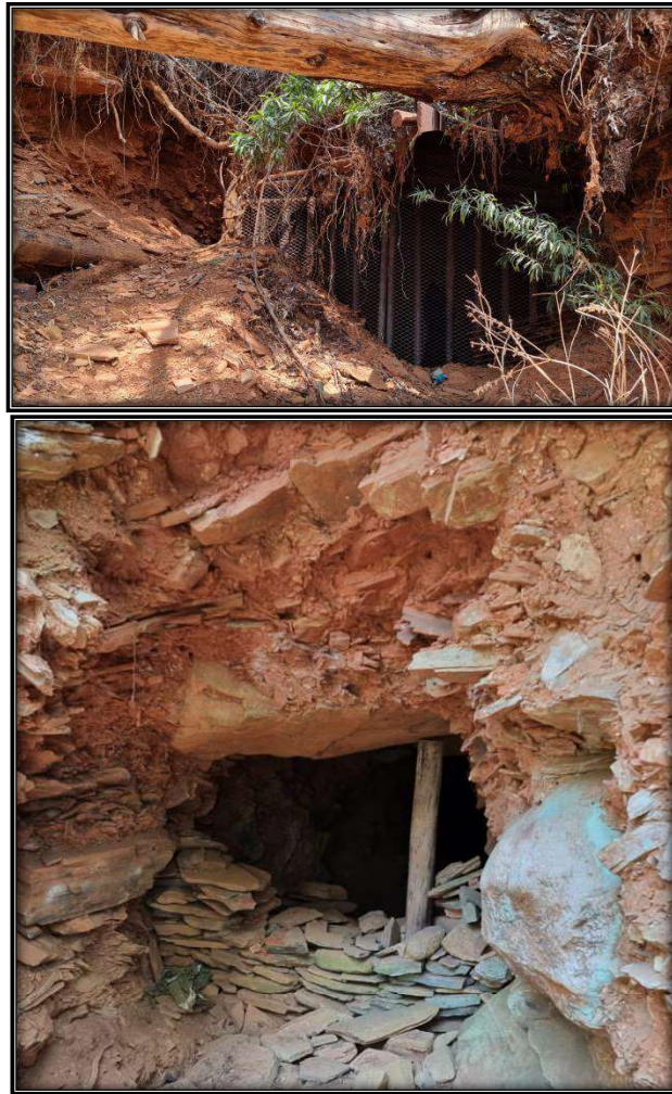
Figure 25: Morgenson Mine Vent shaft
