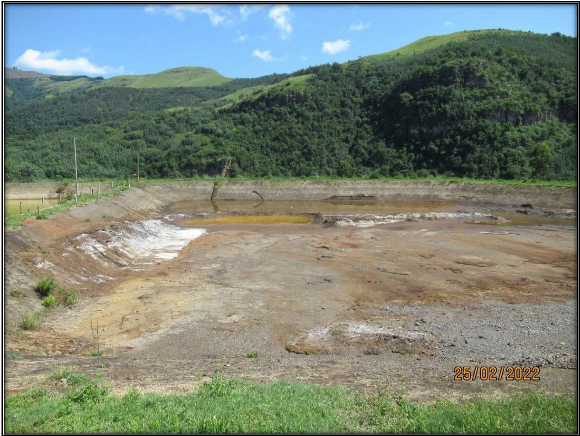
Figure 27: Return Water Dam within dolomite bedrock.
