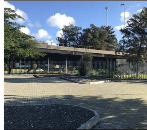
Figure 6A: Highway forms a hostile edge.
