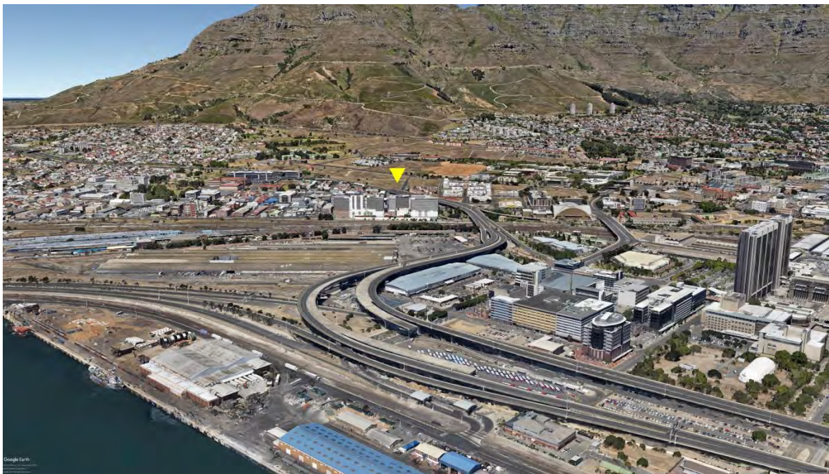
Figure 4.3.5: Birds-eye view of 13 storey proposal looking in a southerly direction over Nelson Mandela Boulevard towards Devil's Peak and Table Mountain. (Google; 2021)
