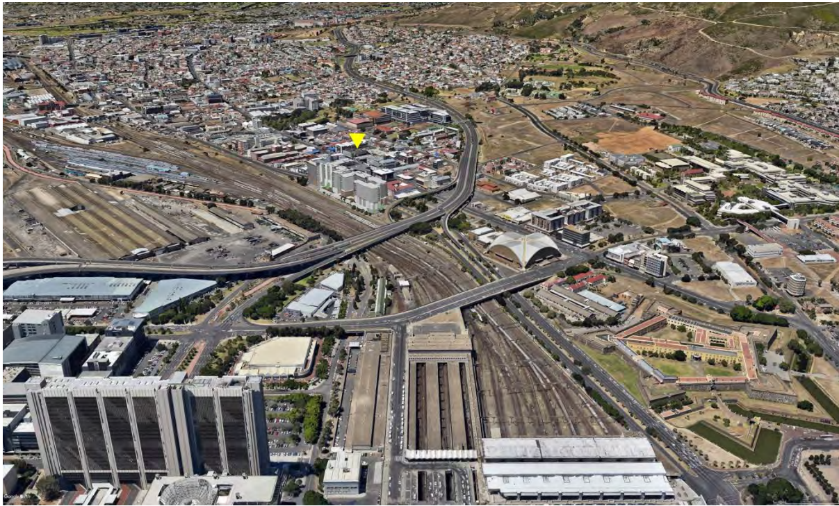
Figure 4.3.4: Birds-eye view of 13 storey proposal from CBD looking towards Woodstock along railway corridor. (Google; 2021)
