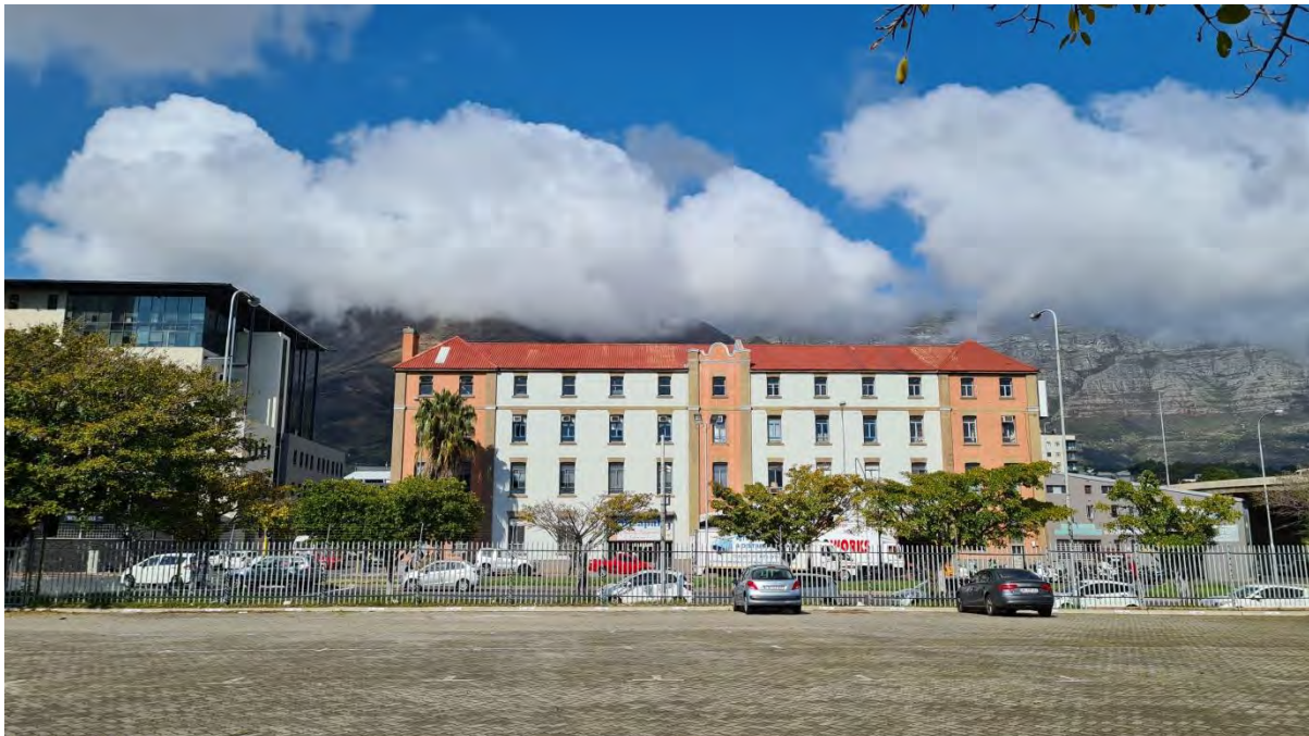
Figure 3.1.1: View from site, looking in a southerly direction towards Devils Peak and Table Mountain (Square One; 2021)
