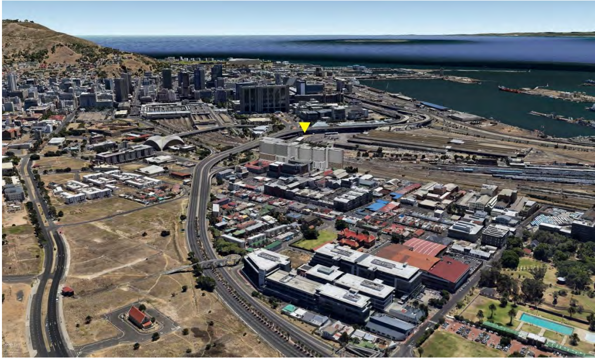
Figure 4.3.2: Birds-eye view of 13 storey proposal from Nelson Mandela Boulevard looking towards the CBD and Cape Town harbour. (Google; 2021)
