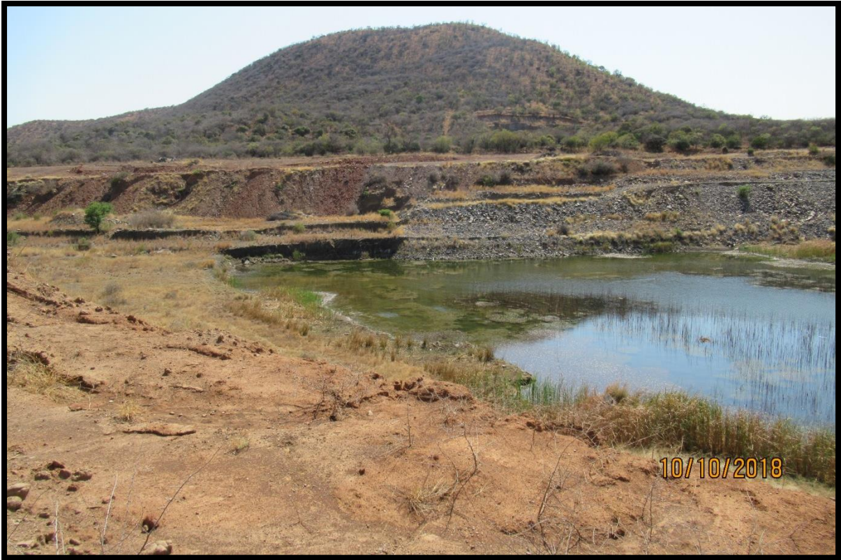
Figure 9: View of remainder of quarry north, rehabilitation has begun.
