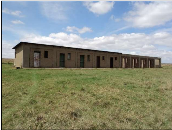
Figure 40: B07 – Modern building.
