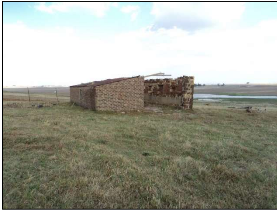
Figure 25: B72 – Building ruin.
