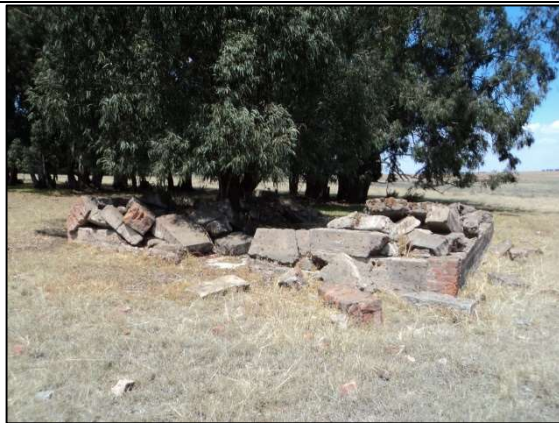
Figure 60: B53 – Building ruin.
