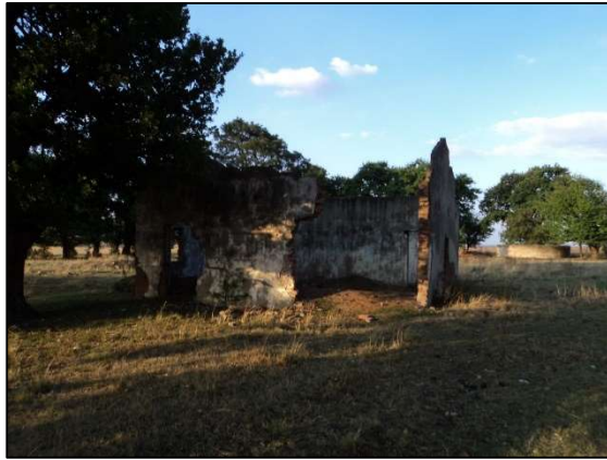
Figure 19: B49 – Building ruin.
