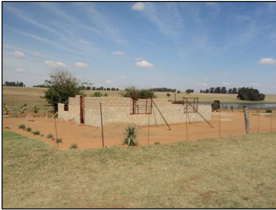
Figure 32: B05 – Modern building.
