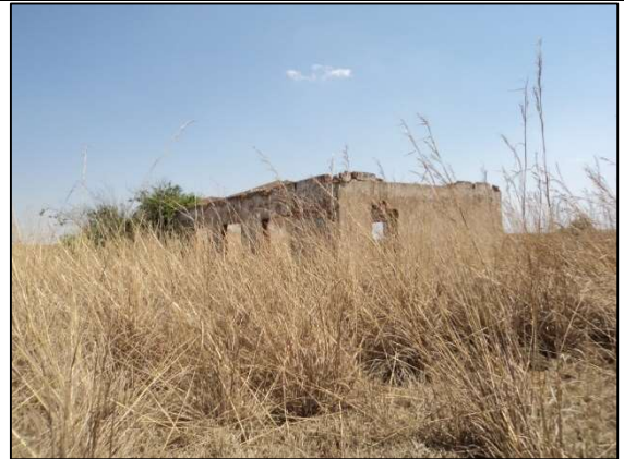
Figure 43: B12 – Building Ruin.
