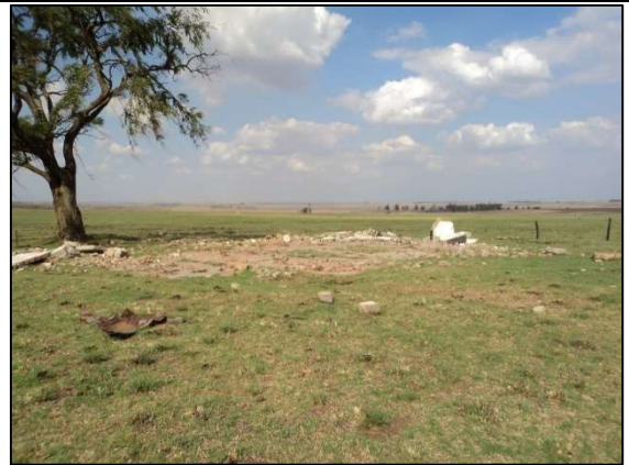
Figure 59: B44 – Demolished building.
