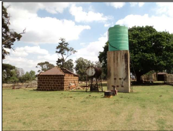
Figure 48: B22 – Outbuilding & water tank.
