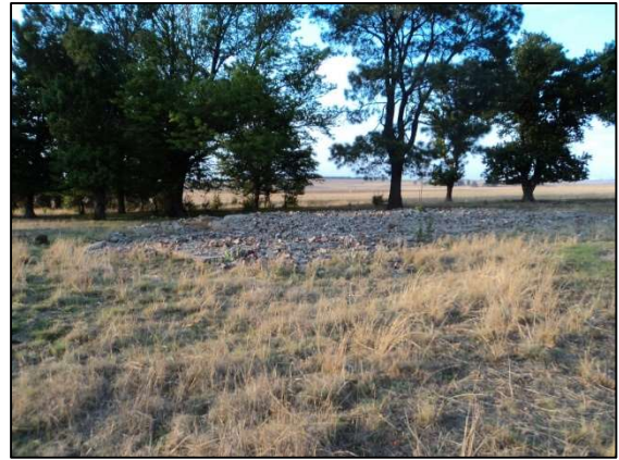
Figure 20: B49 – Demolished building.
