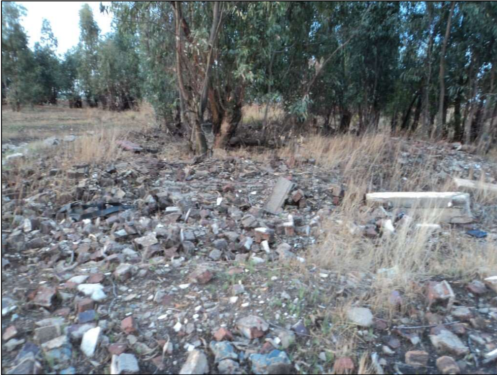
Figure 21: Building rubble at Site BA02.
