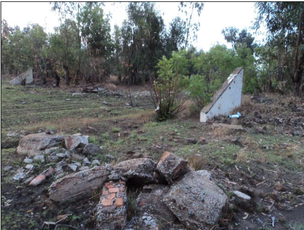
Figure 22: General condition of structures associated with Site BA02.
