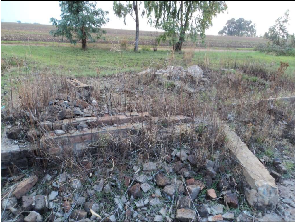
Figure 23: Foundation remains at Site BA02.
