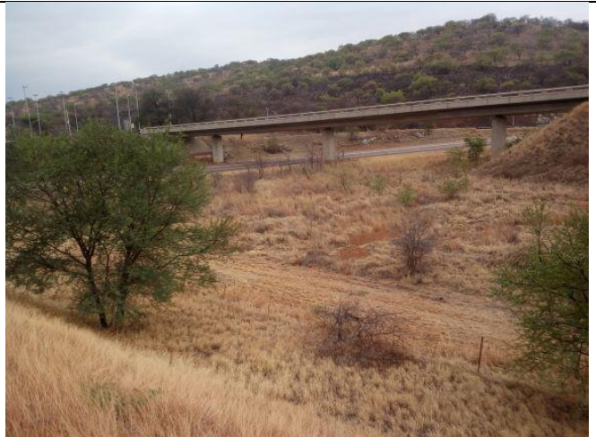
Fig 2. View of ramp area
