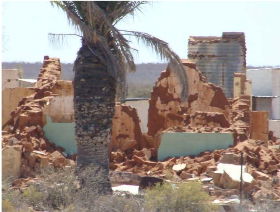
Figure 47 Partially demolished building at site no. 24.
