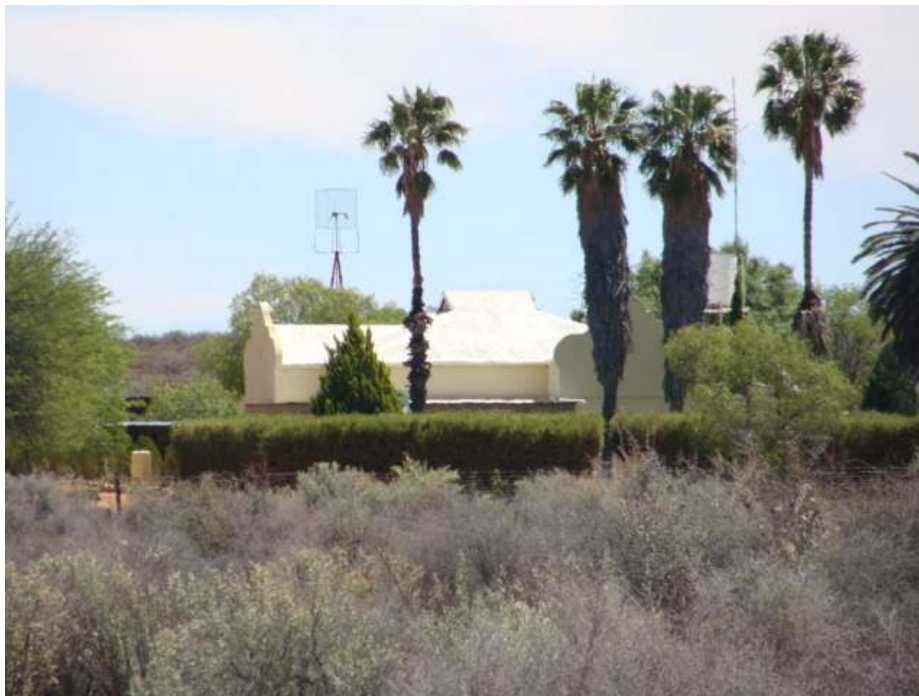
Figure 28 Main house, unfortunately hid by a fence, at site no. 9.
