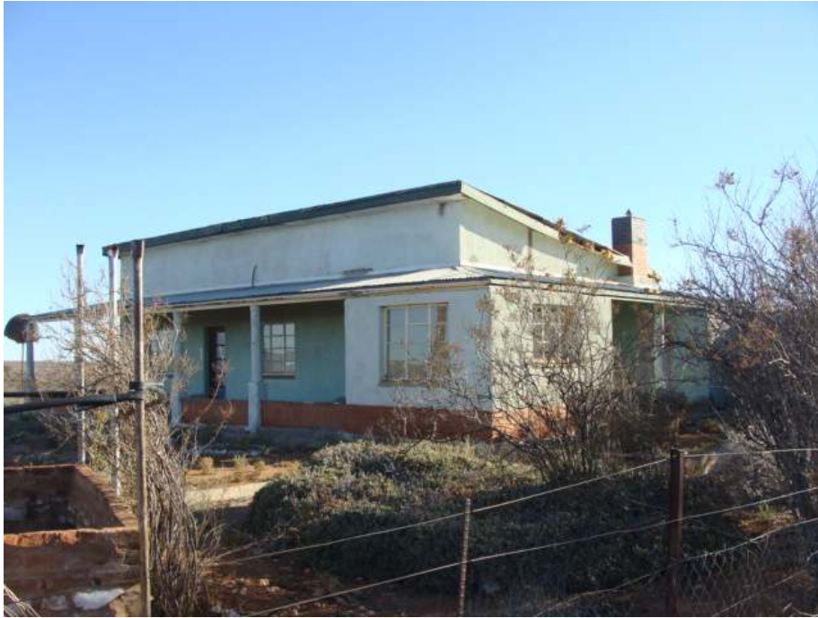
Figure 44 Main house at site no. 23.
