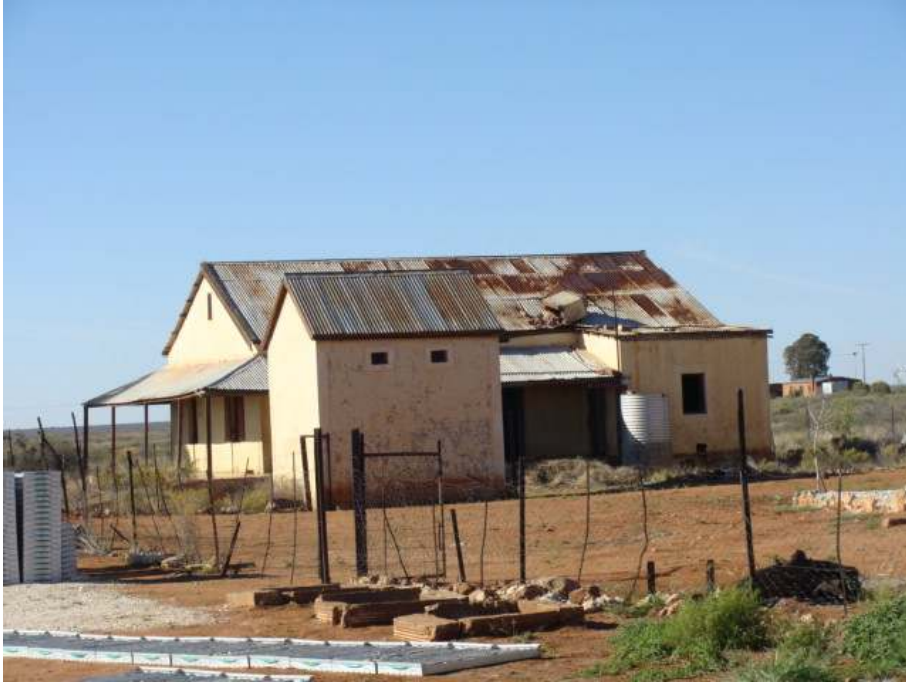
Figure 55 The new police station and jail at Putsonderwater.
