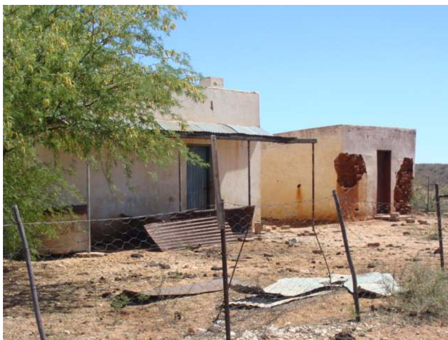
Figure 21 Buildings at site no. 5.
