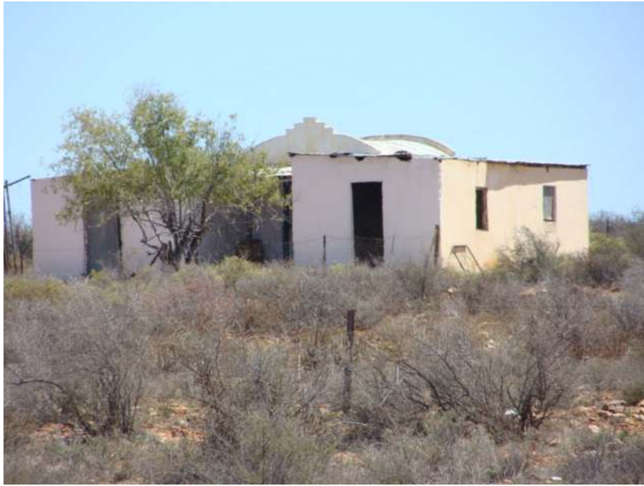
Figure 30 Buildings at site no. 11.
