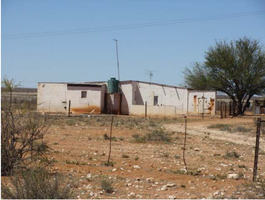
Figure 38 Main house at site no. 18.
