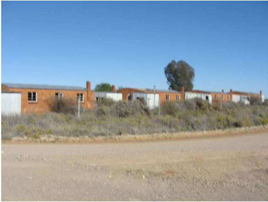
Figure 51 Railway houses at the Putsonderwater station.
