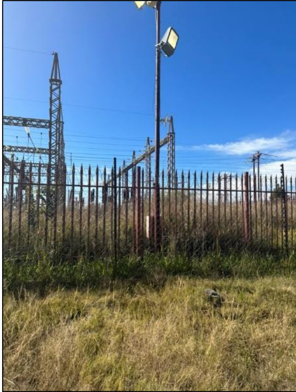
Figure 4 – View of reclamation pump stations at the most western end of the pipeline .
