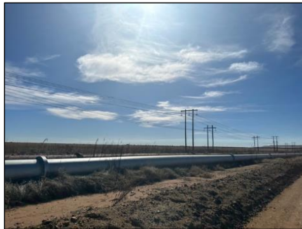
Figure 7 – View of existing pipeline.
