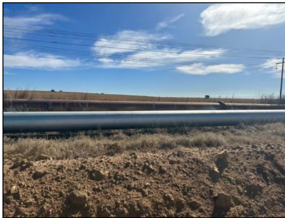
Figure 6 – View of existing pipeline.
