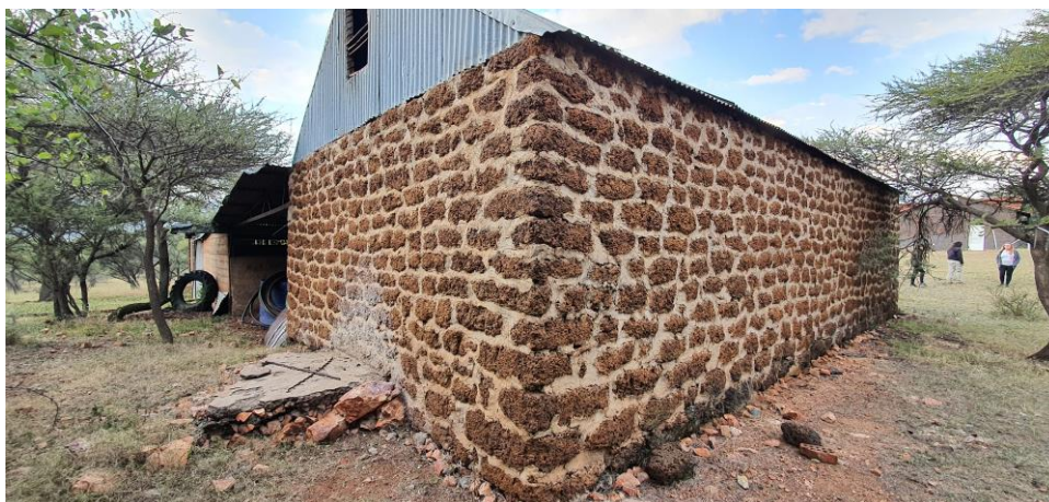
Figure 38: The shed constructed from dressed ferricrete rocks
