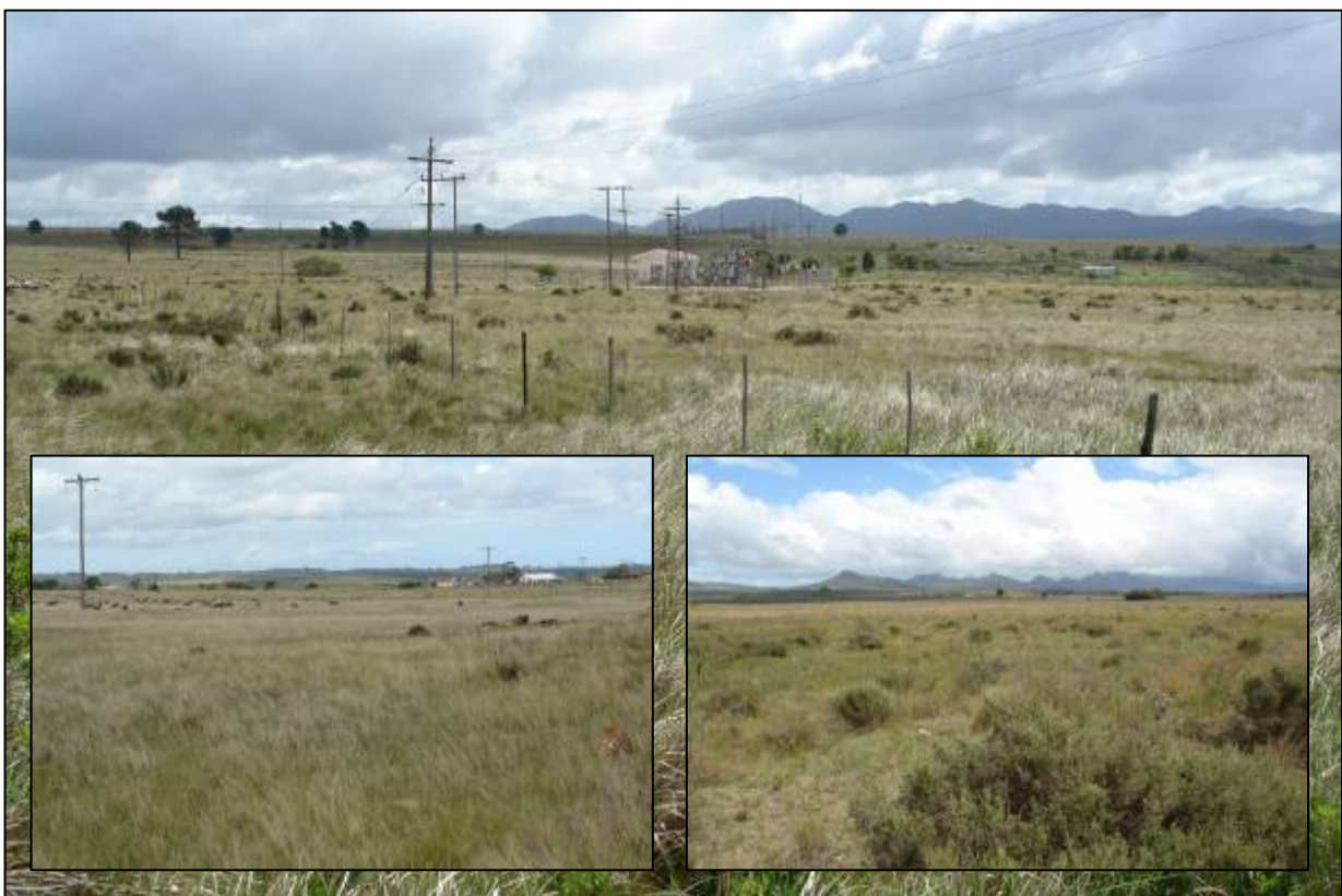
Fig. 9. General views of the existing Dieprivier Substation and the surrounding landscape.
