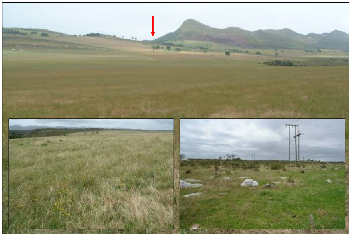
Figure 5. General views of the line route from the hill crossing (red arrow) towards the Krom River (main image and left insert) where it joins the original line route (right insert) towards the Dieprivier substation.
