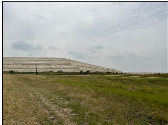
Figure 11 – View of existing TSF.
