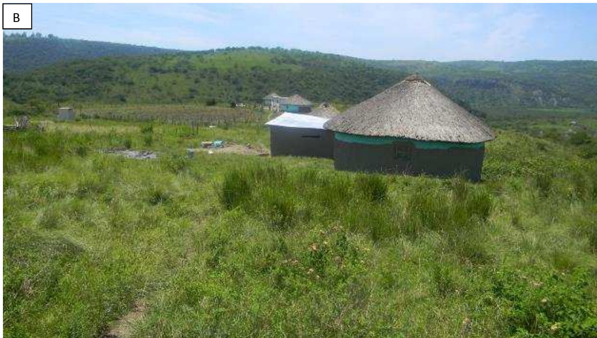
Figure 7 B: View of some homesteads at Egoli Village, LV lines will be connected to homesteads such as this one. The impact of LV lines is very limited
