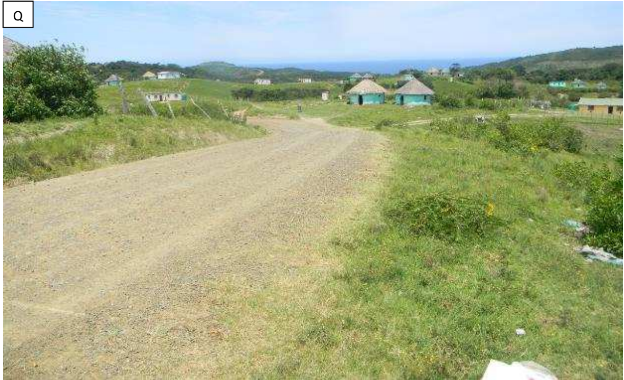
Figure 22 Q: View of located along road servitude at Mdzweni village. The MV line will run along road servitude while LV lines will branch to homesteads.
