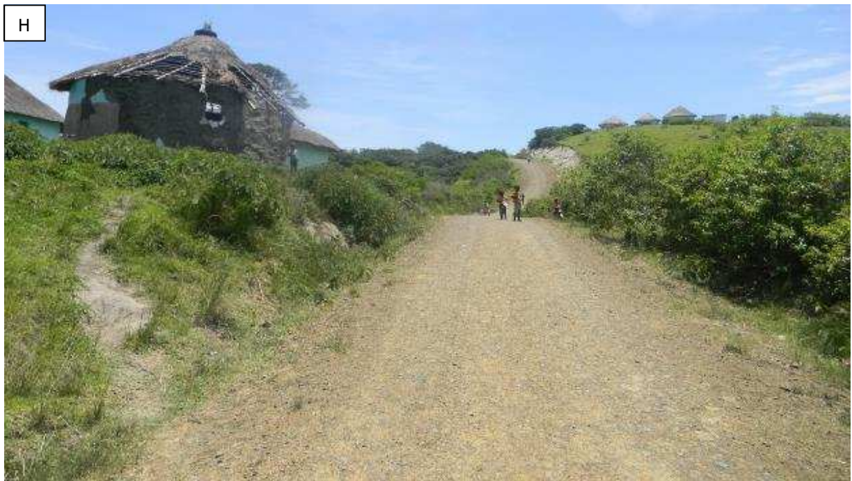
Figure 13 H: View of power line route along roads servitude
