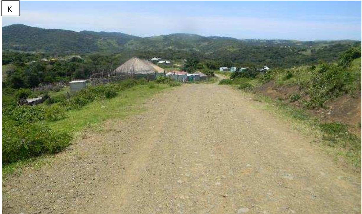
Figure 16 K: View of homesteads located along road servitude. Note that the power line route will run along the road reserve and LV lines will branch to individual homesteads.
