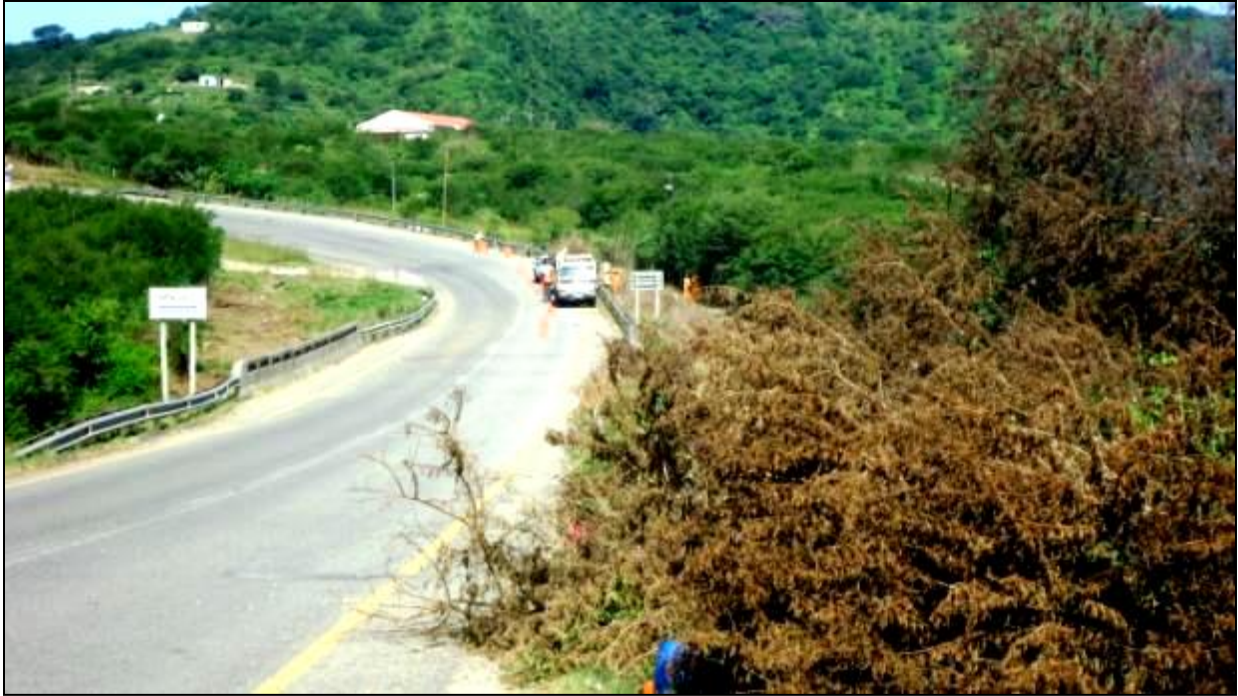
Fig 23 Bridge over Mngazi River on R 61 Dead, cleared growth in foreground
