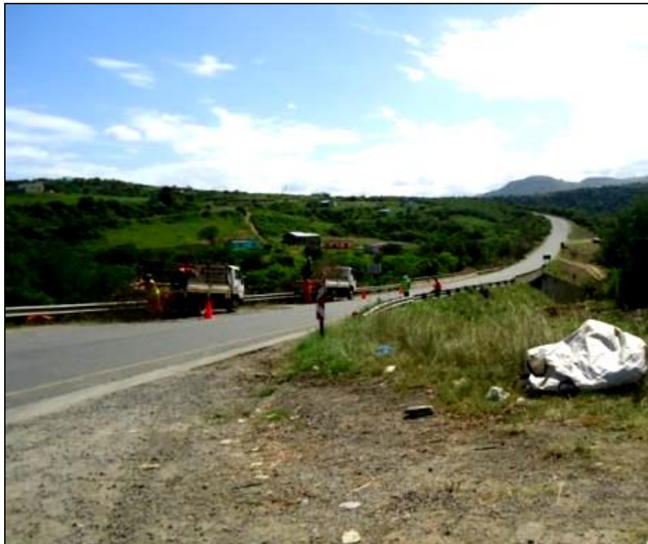
Fig 14 R61 Mngazi River Bridge looking towards Mthatha
