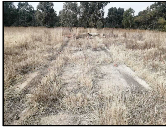
Figure 8.3. Cement foundations at KE001.
