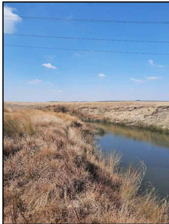
Figure 7.4. General site conditions where the existing powerlines cross the river.
