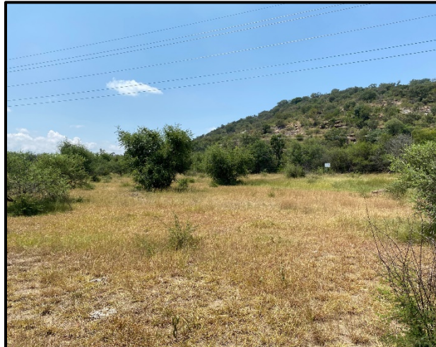
Figure 7.2. Existing powerlines in the area.
