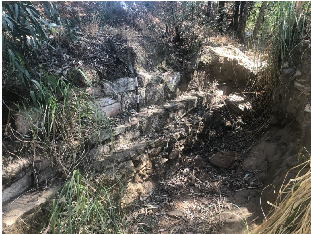
Figure 27 – Exposed stone walling at VS1
