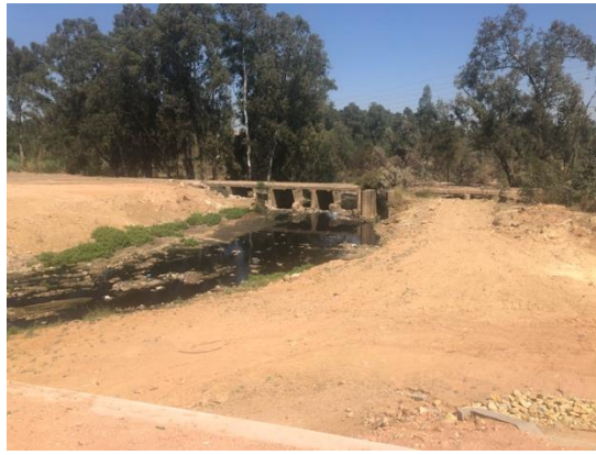
Figure 8 - View of old Crownwood road bridge
