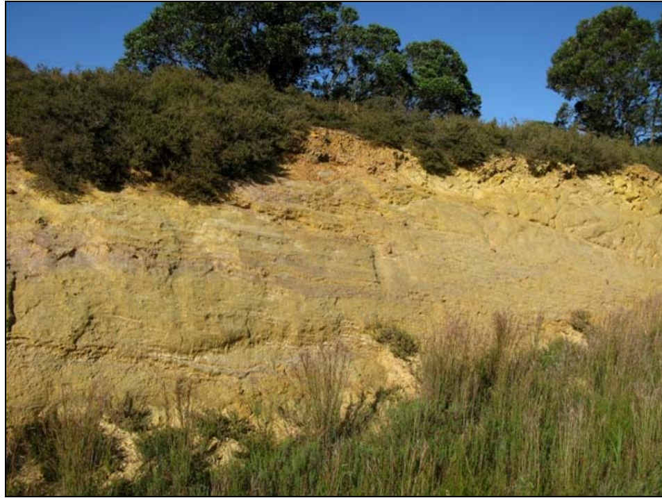
Figure 7. Deeply-weathered saprolite developed from thin-bedded mudrocks of the Gydo Formation, N-facing roadcut on the N2 (Loc. 149).
