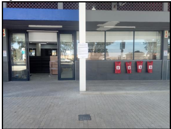
Figure 3.4. Current site conditions
