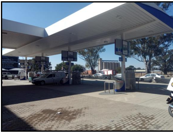
Figure 3.1. Current site conditions
