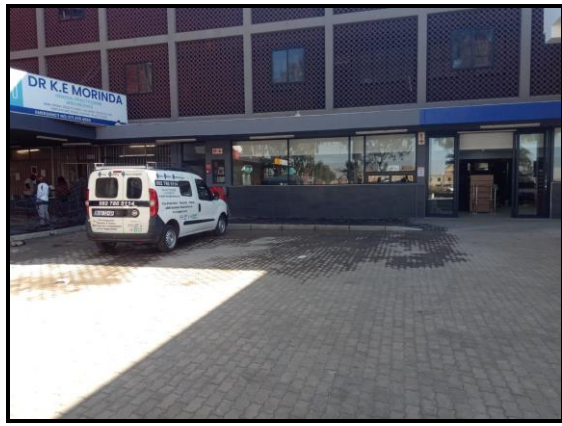
Figure 3.2. Current site conditions
